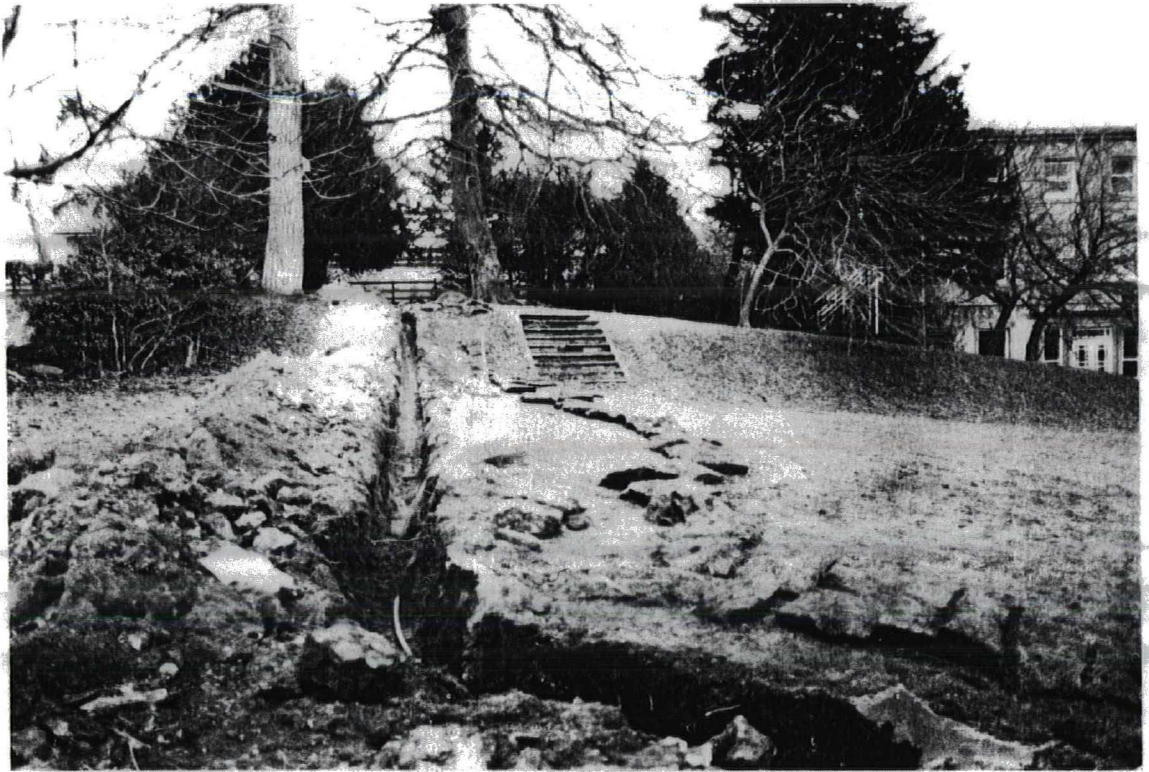
Plate 1. General view of pipe trench. Facing north.
