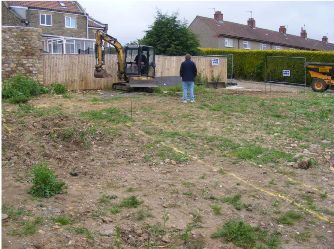
Plate 1. Pre-Excavation Shot. Facing North-West
