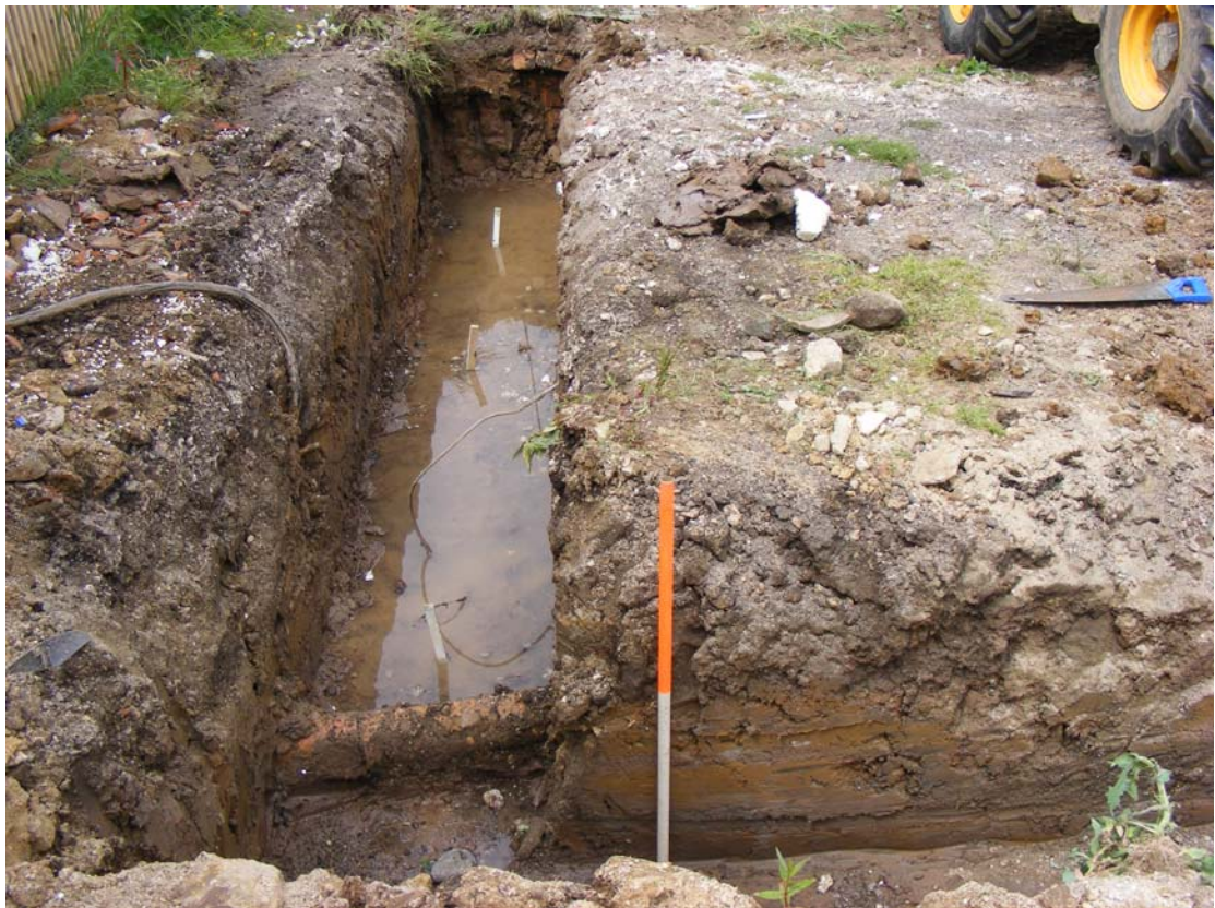
Plate 2. Foundation Trench and Drain. Facing North
