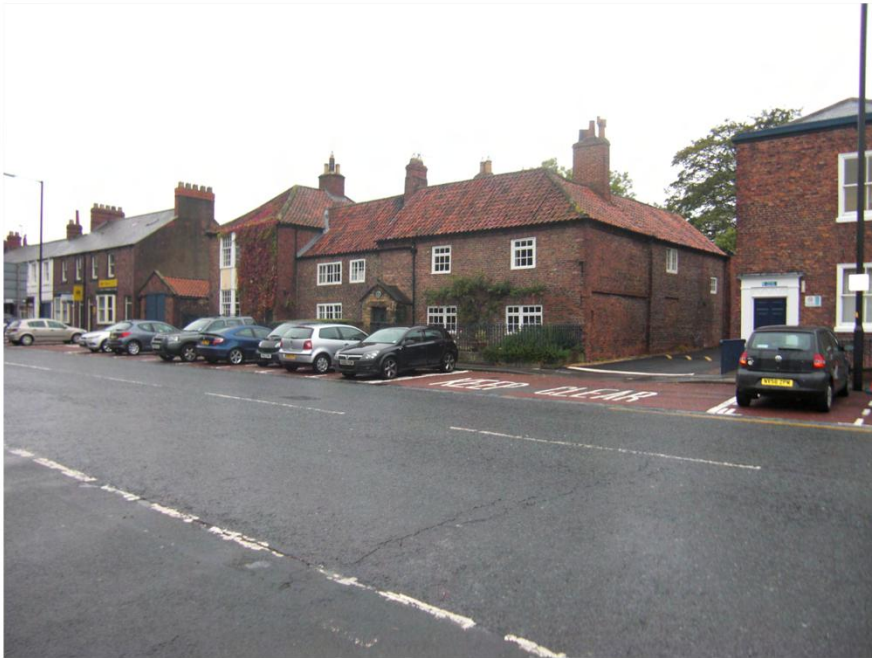
Plate 1. Porch House, Northallerton. Facing North-east.
