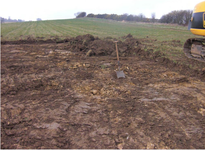
Plate 5. Area of Topsoil Stripping. Facing South-west.
