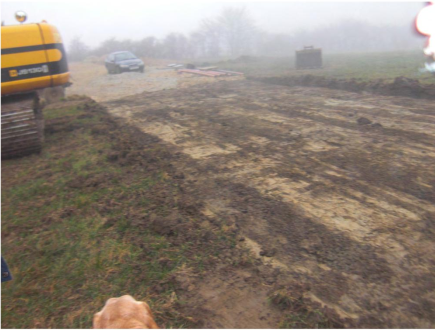
Plate 1. Area of Topsoil Stripping. Facing North-west.
