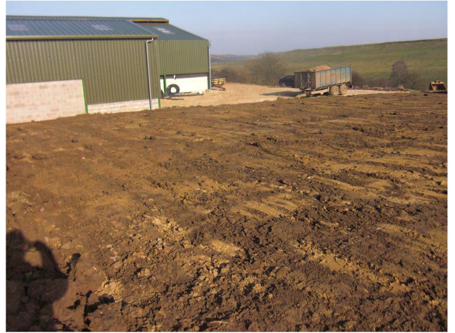
Plate 4. Area of Topsoil Stripping. Facing North
