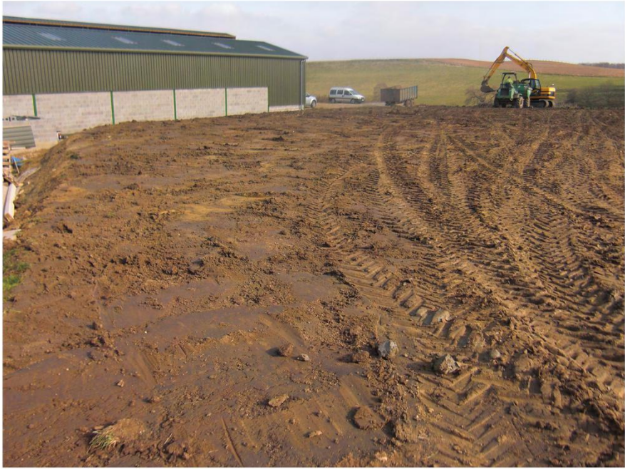
Plate 6. Area of Topsoil Stripping. Facing North-east.
