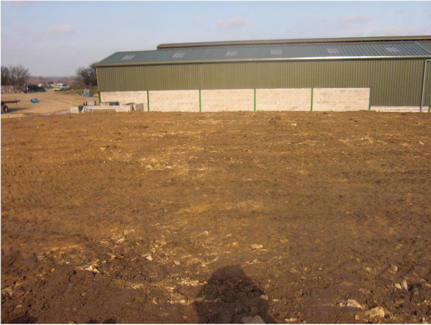
Plate 7. Area of Topsoil Stripping. Facing North.
