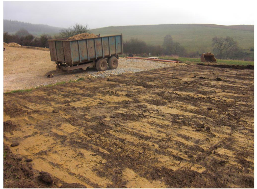
Plate 2. Area of Topsoil Stripping. Facing North.
