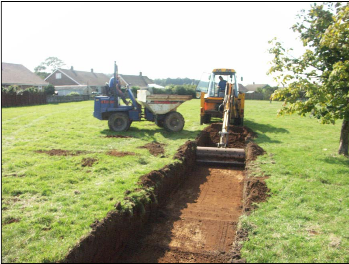
Figure 3 Stripping the site by machine
