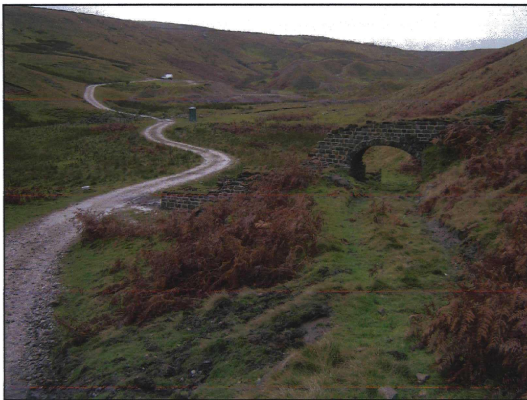
Plate 4. East side of arch over track-way after works, looking west.
