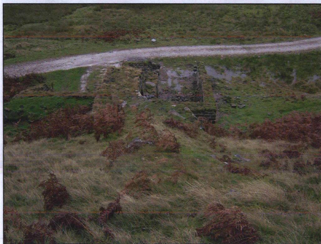
Plate 6. Looking south along the line of the flues, after works.
