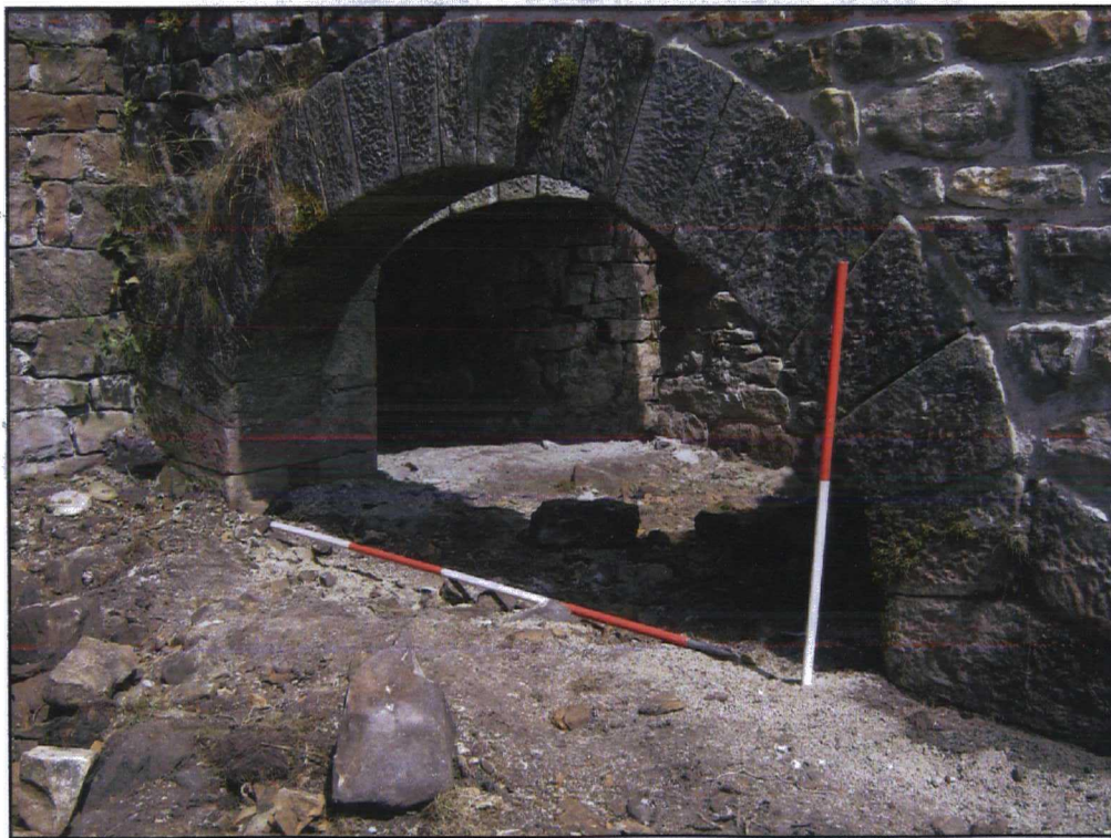
Plate 10. Archway in Room 1 looking north-east during works. Scales 1&2m.
