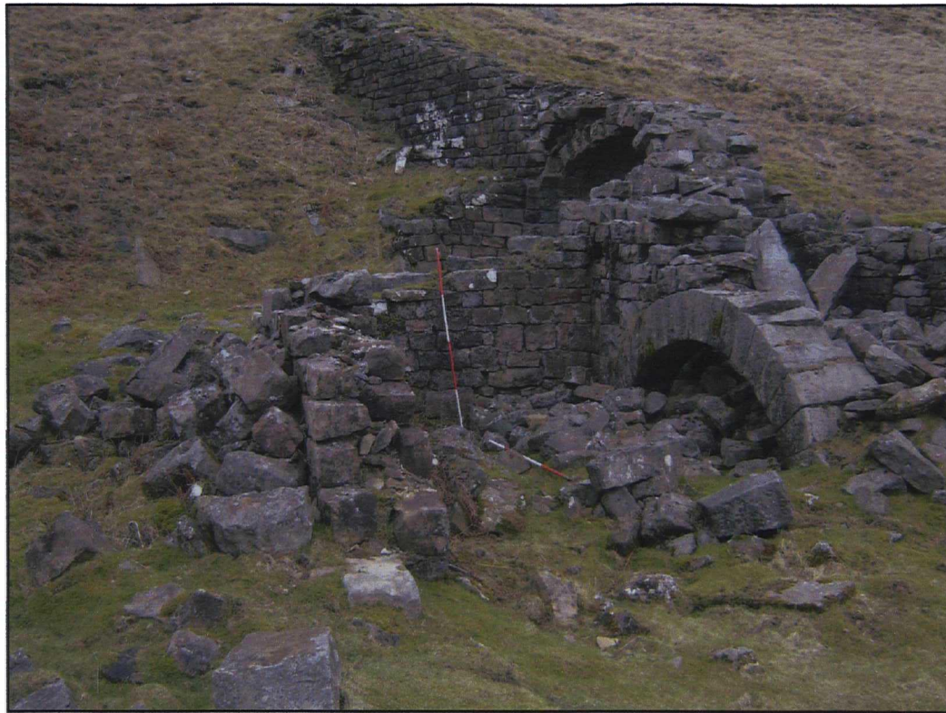
Plate 7. General view of Room 1, looking north-east before works, scales 2m.
