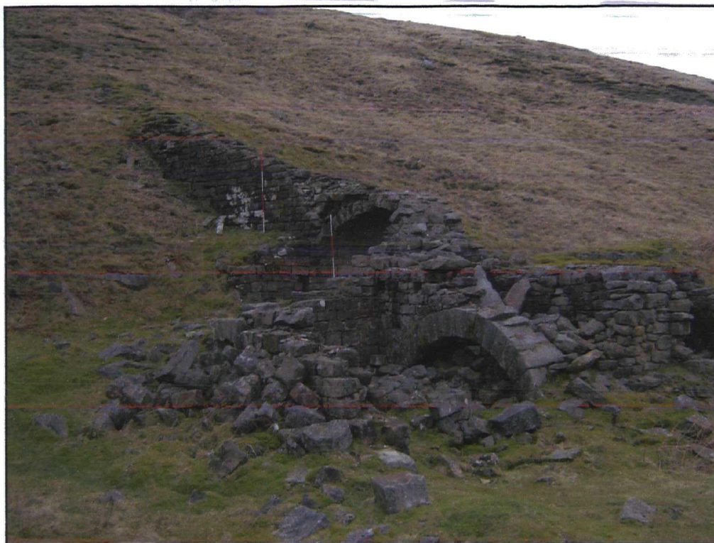
Plate 1. General shot of smelt mill, looking north-east before works, scales 2m.
