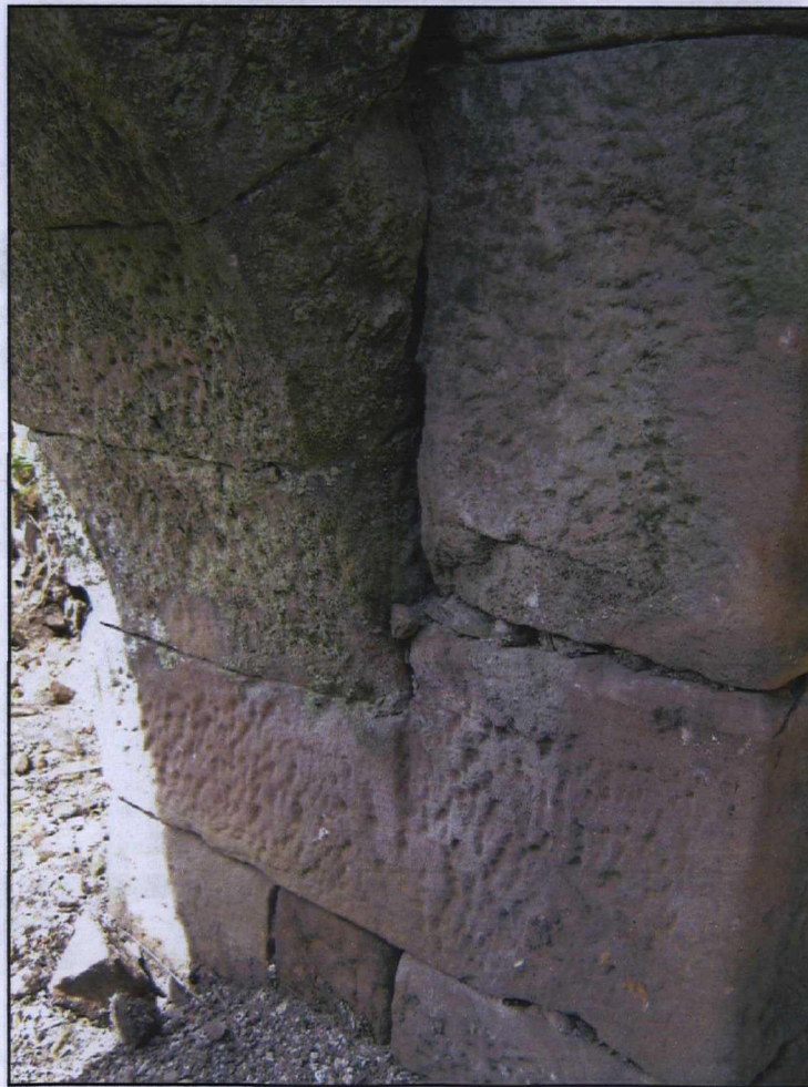
Plate 12. Spring point for northern end of arch in Room 1, looking north-west.
