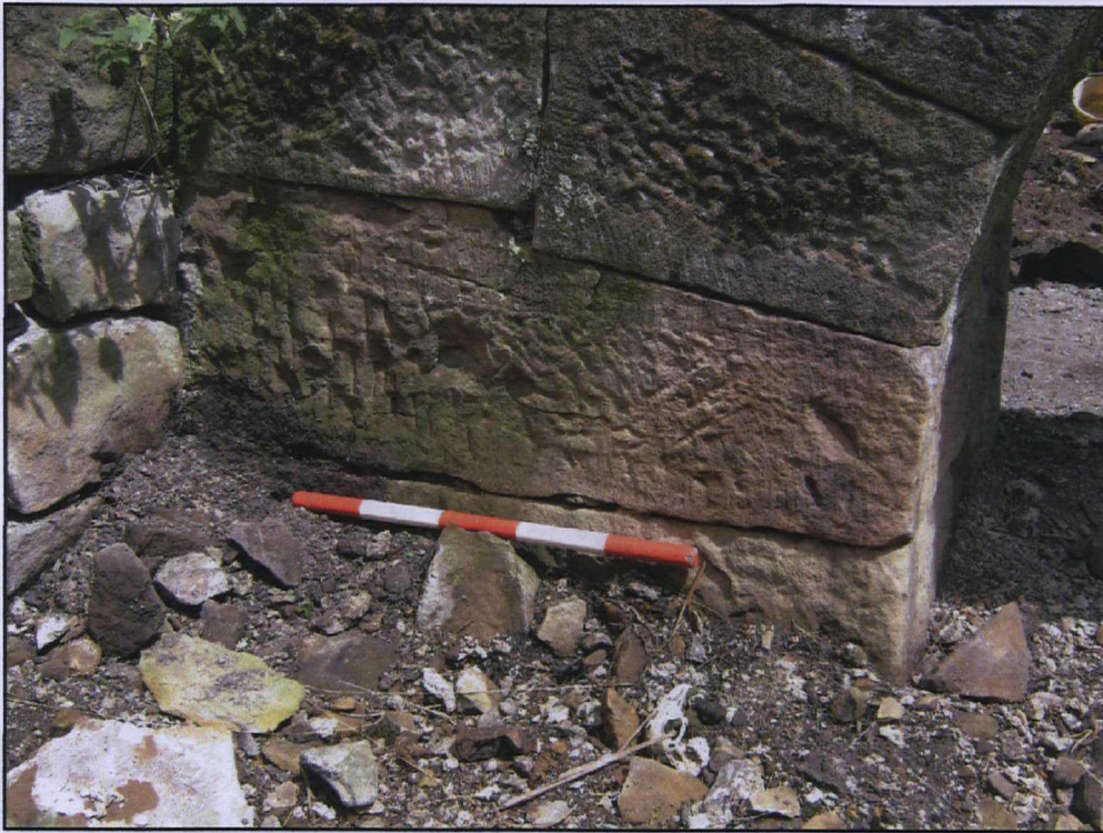
Plate 11. Spring point for northern end of arch in Room 1, looking east. Scale 0.5m.
