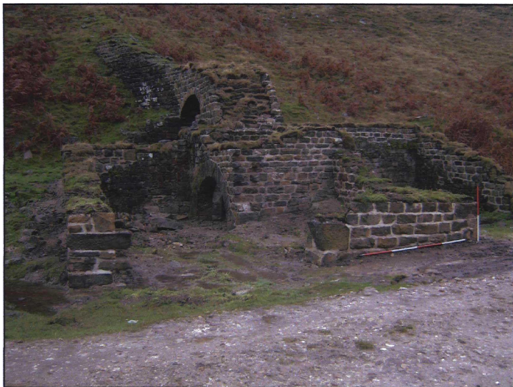
Plate 8. General view of Room 1, looking north-east after works, scales 1&2m.
