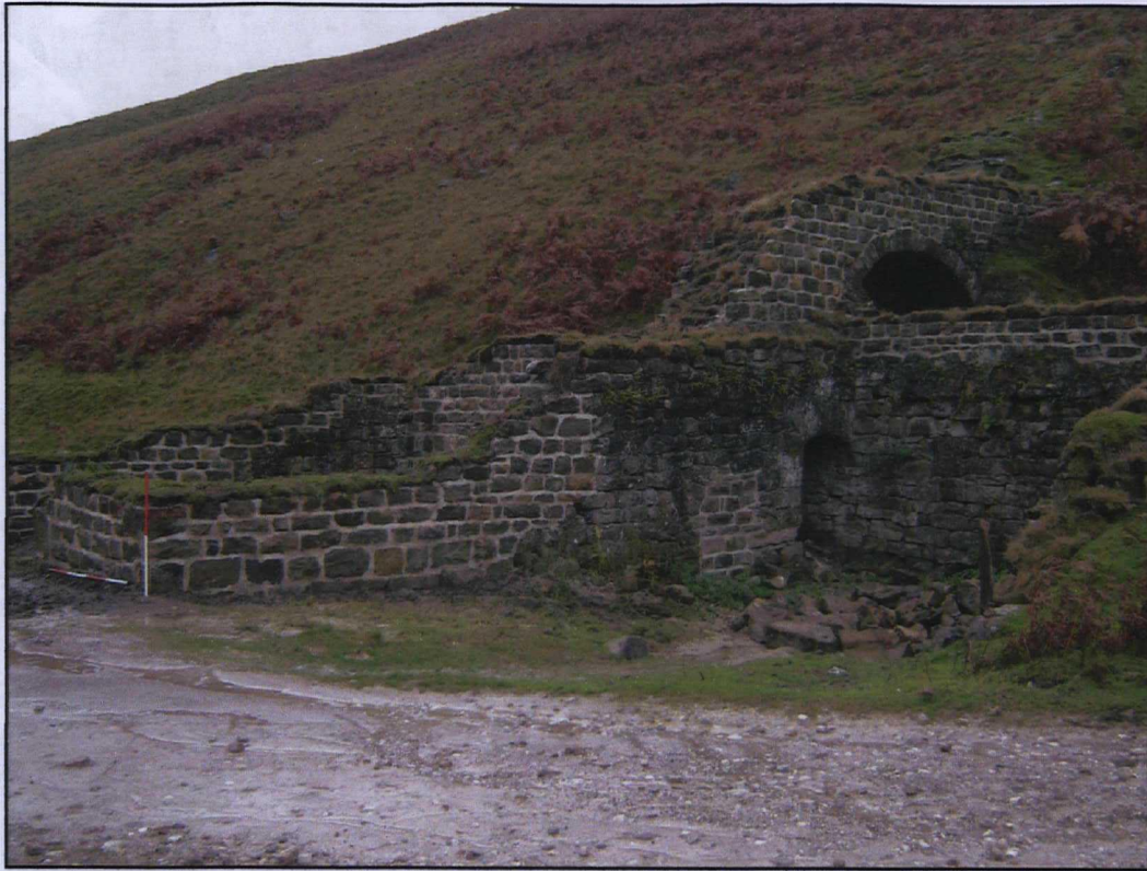
Plate 27. Room 5 after works, looking north-west. Scales 1&2m.
