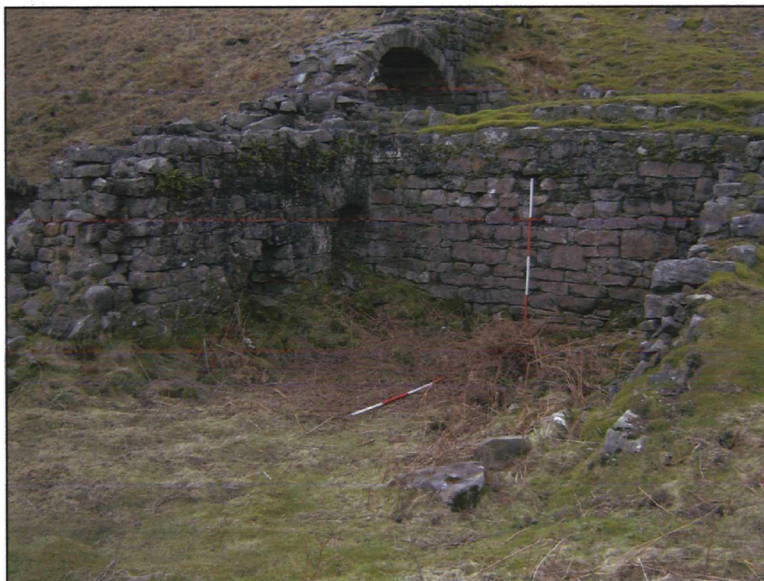
Plate 26. General view of Room 5 before works, looking north-west, scales 2m.
