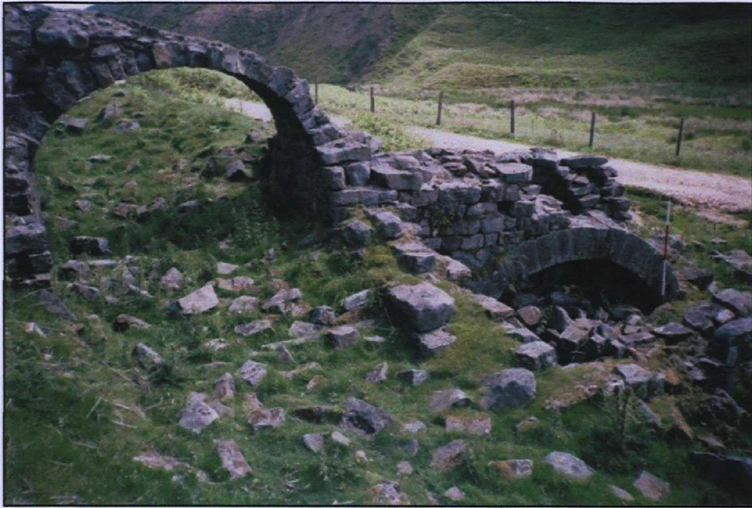
Plate 32. Providence Smelt Mill Flue (M Roe, 2003)
