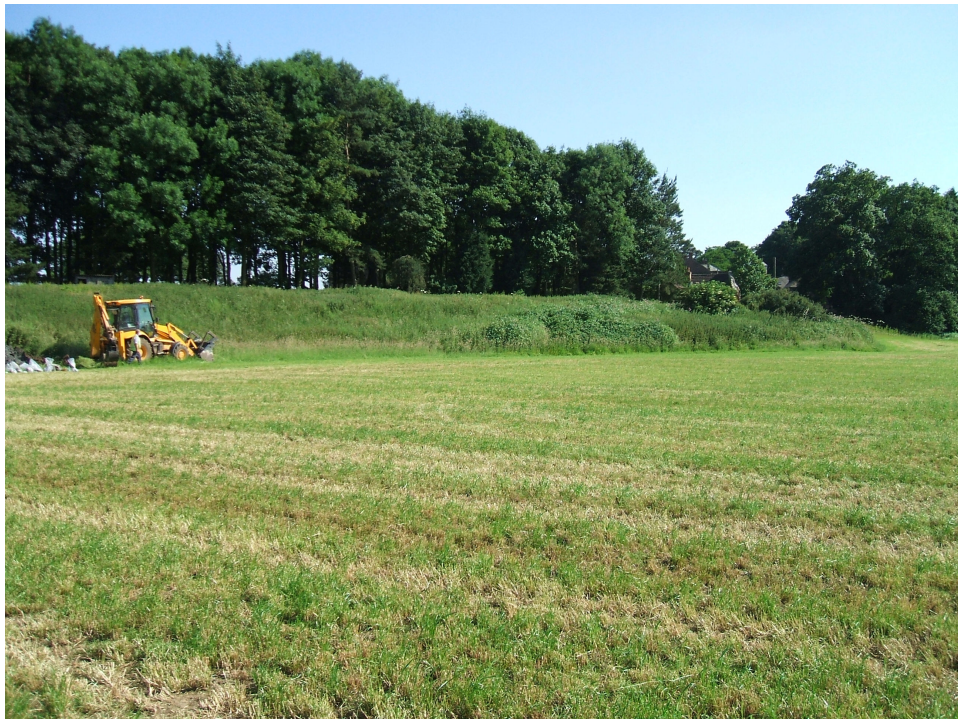
Plate 4 TPSA 005 looking east. Flood plain (foreground), terrace (background), Brawith Hall behind trees (right)
