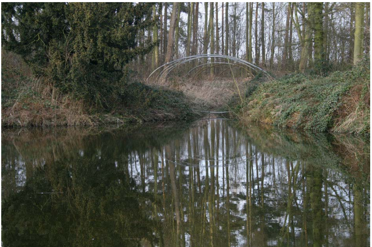
Plate 20: Site 01 , north-east pipe, looking north-east
