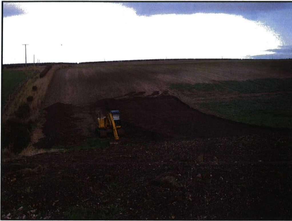
Plate 1: The topsoil strip, view north-east
