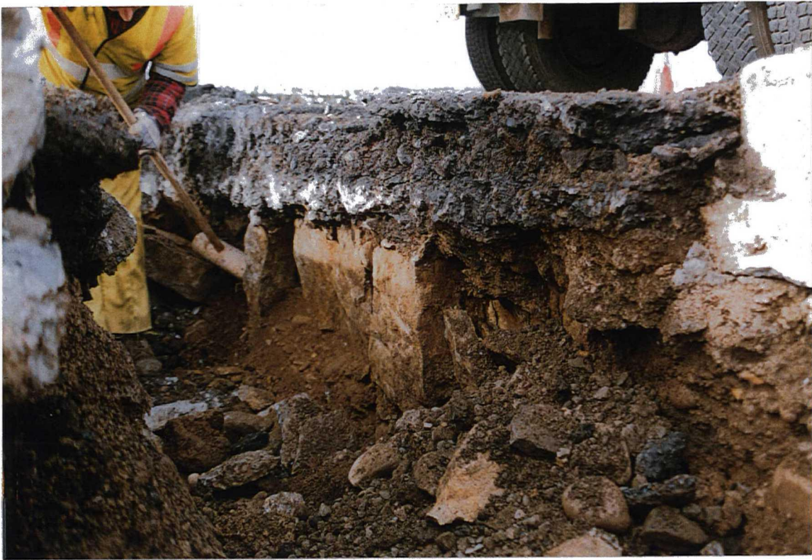
PLATES 5 & 6 ROAD CROSSING SHOWING STONE BASE BELOW CONCRETE AND TARMAC SURFACE
