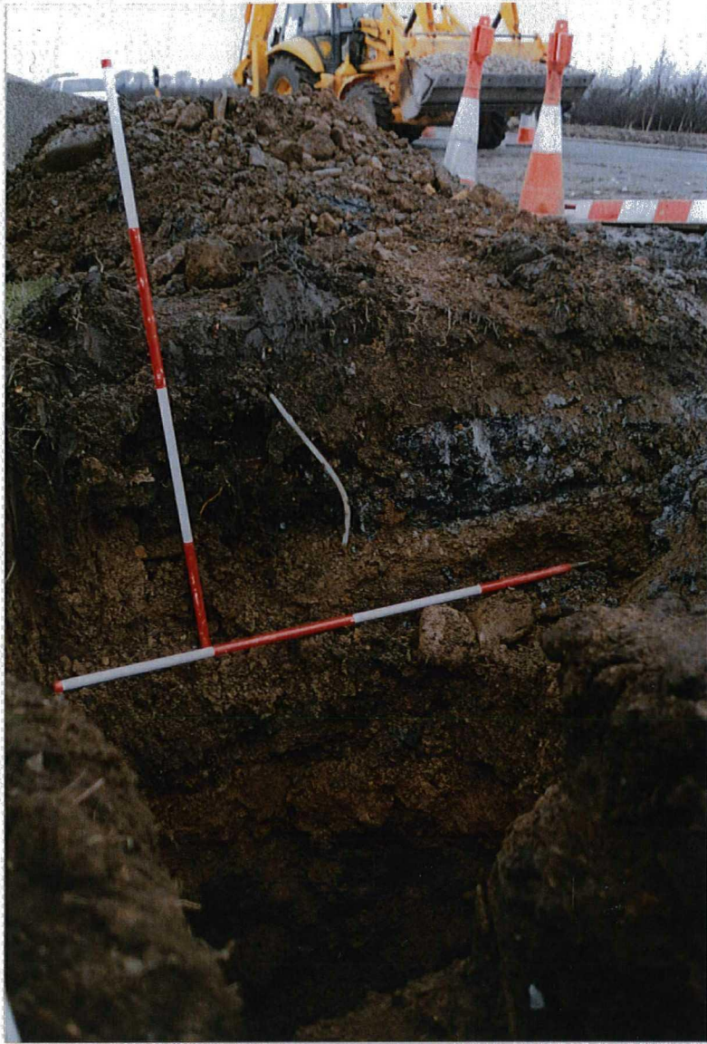
PLATE 1 SOAKAWAY IN TRENCH 3, SHOWING FORMER ROAD SURFACES AND LAYERS OF GRAVEL AND SILTS
