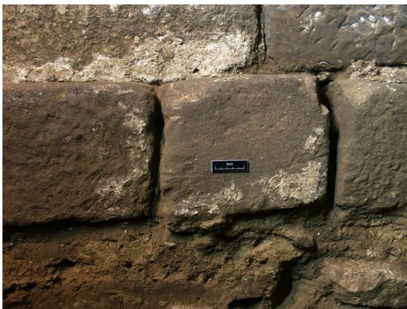
Plate 8 Plaster/ render on side of reused gritstone blocks
