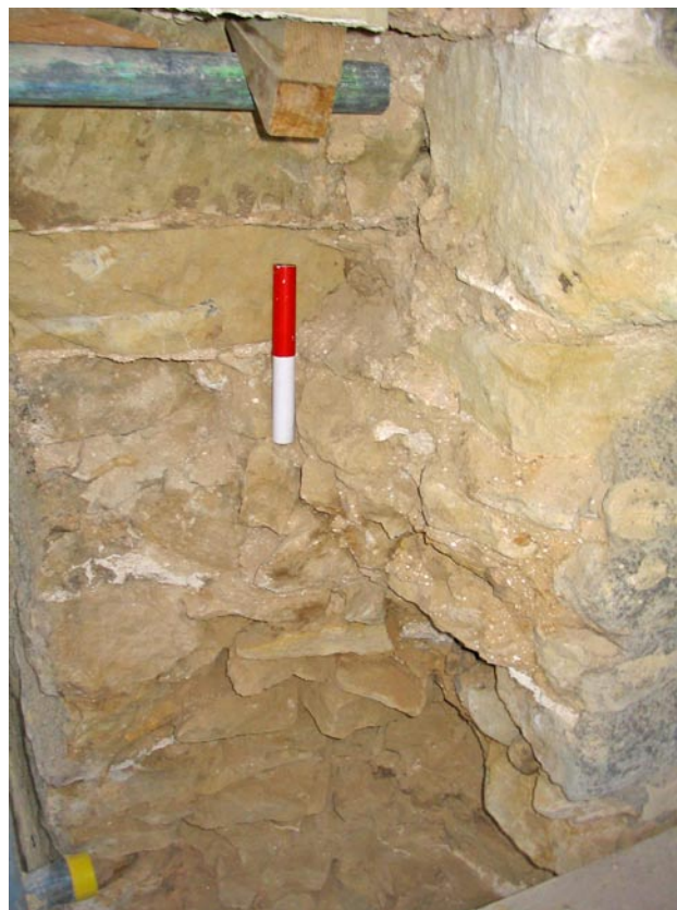
Plate 44 Mortar working phases in tower core
