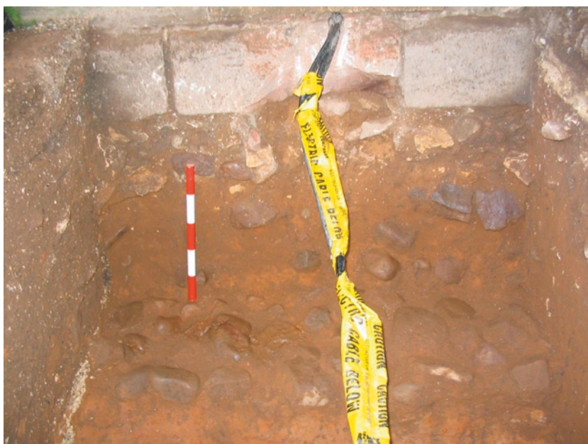
Plate 24 Rubble foundations for standing building overlying cobble foundations for earlier structure
