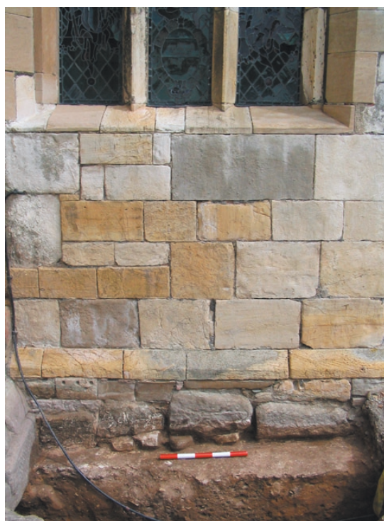
Plate 37 Rebuilt western wall of the southern aisle
