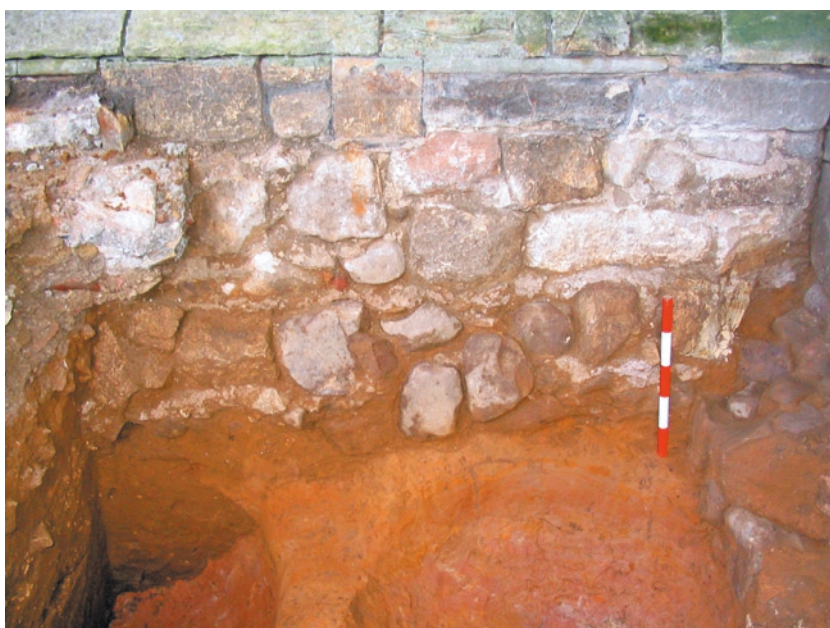
Plate 35 Western wall and foundation of northern aisle
