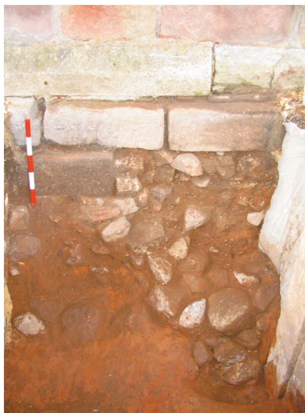
Plate 28 The gritstone block and rubble foundations for standing tower, over the earlier cobble foundations at the south of the tower
