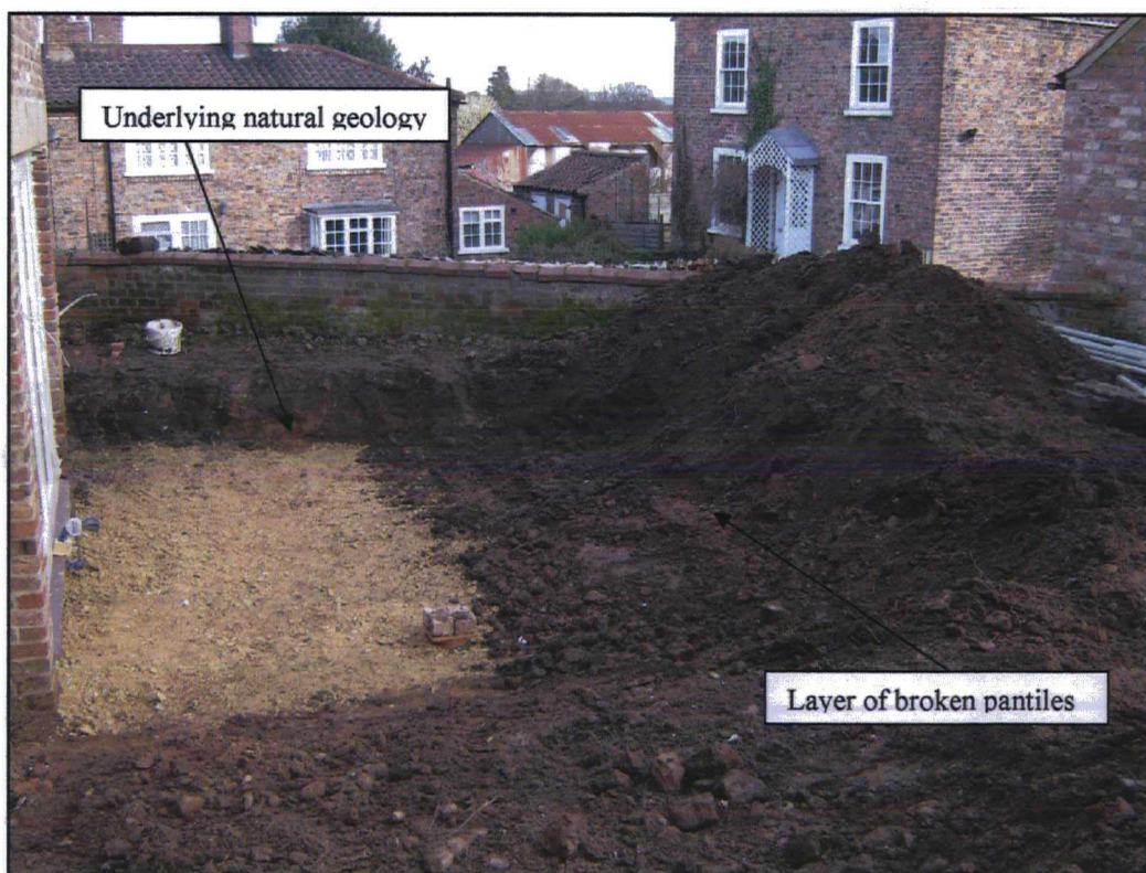
Plate 2. Looking north-east showing ground reduction to east of barn.
