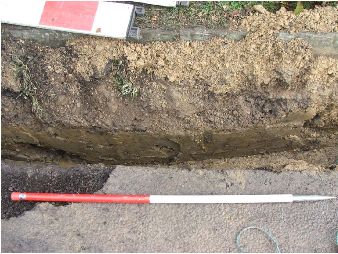
Figure 3 The service trench looking south
