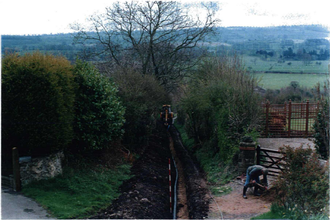
North / Central section of service trench, facing south.
