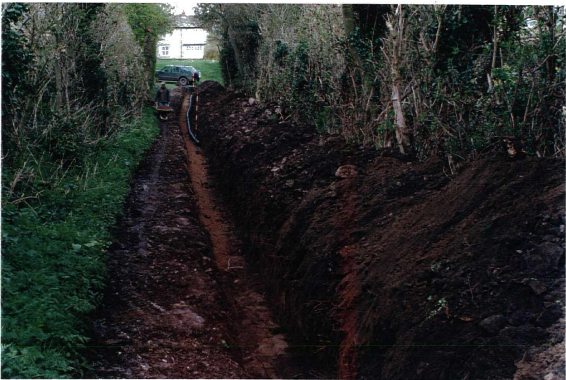
Central / North section of service trench, facing north.
