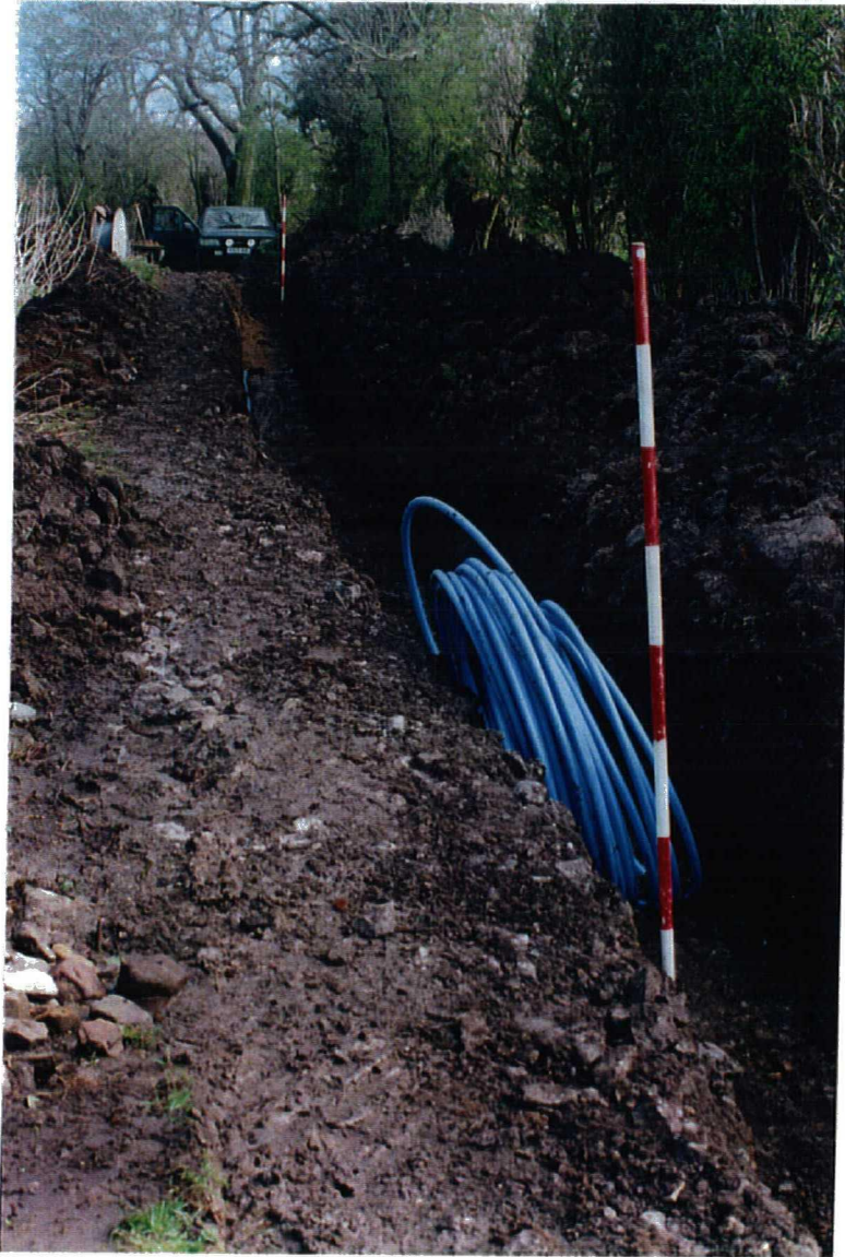
Southern section of service trench, facing north north east.
