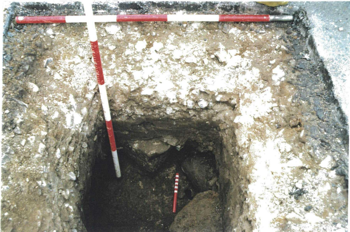
Trial Hole No.3, detailing rubble fill and mortar crust.
