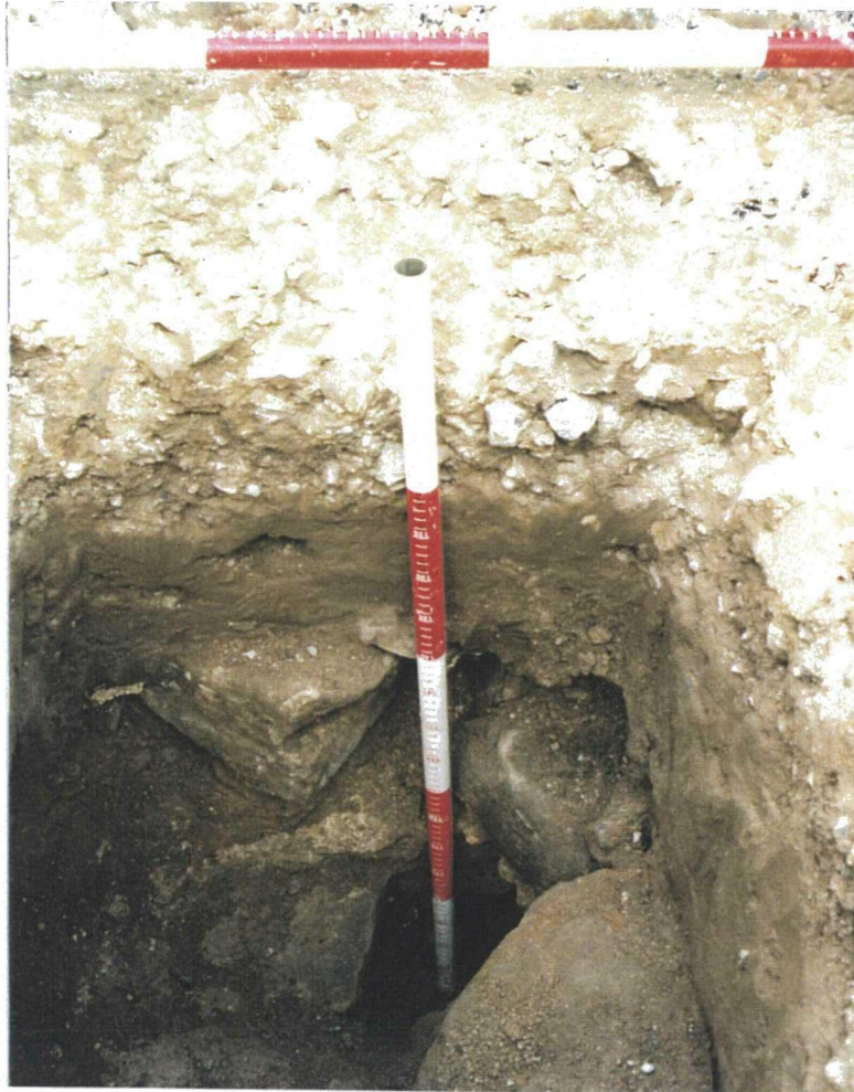
Trial Hole No.3, detailing mortar crust and void onto arch ring.
