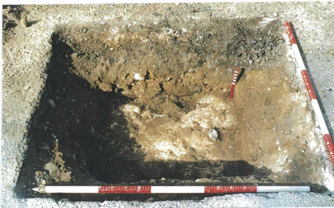
Trial Hole No.3, detailing fill of pier.
