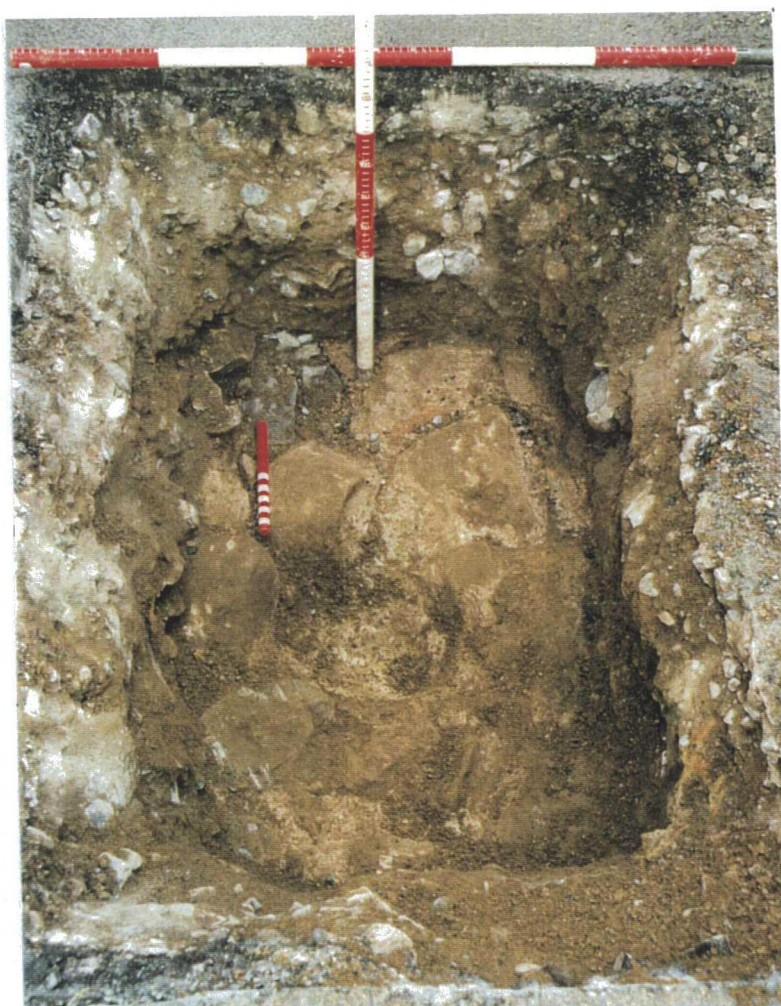
Trial Hole No.2, detailing fill of pier.
