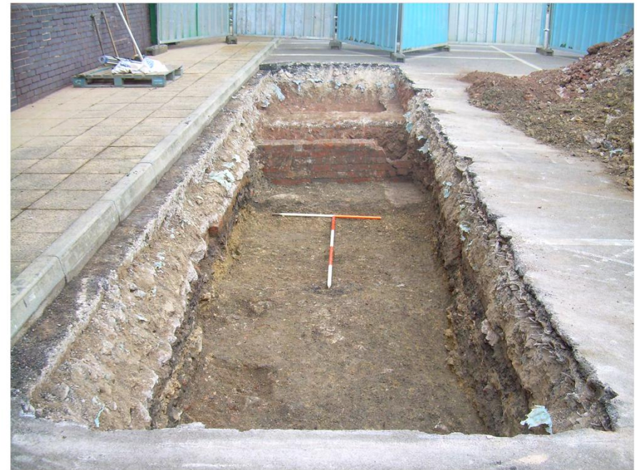
Plate 2. View of Trench 1 after cleaning. Facing East.
