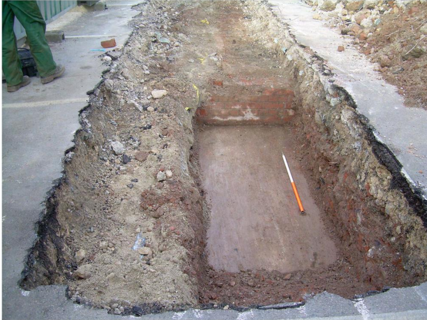
Plate 9. Trench 2: Concrete Floor 2019. Facing West.
