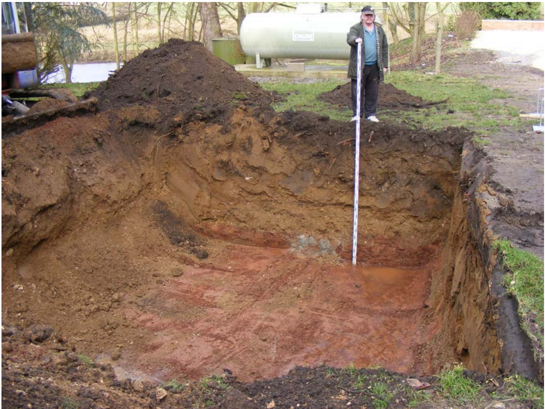
Plate 2 Post-Excavation shot of Gas Tank Pit. Facing North-West
