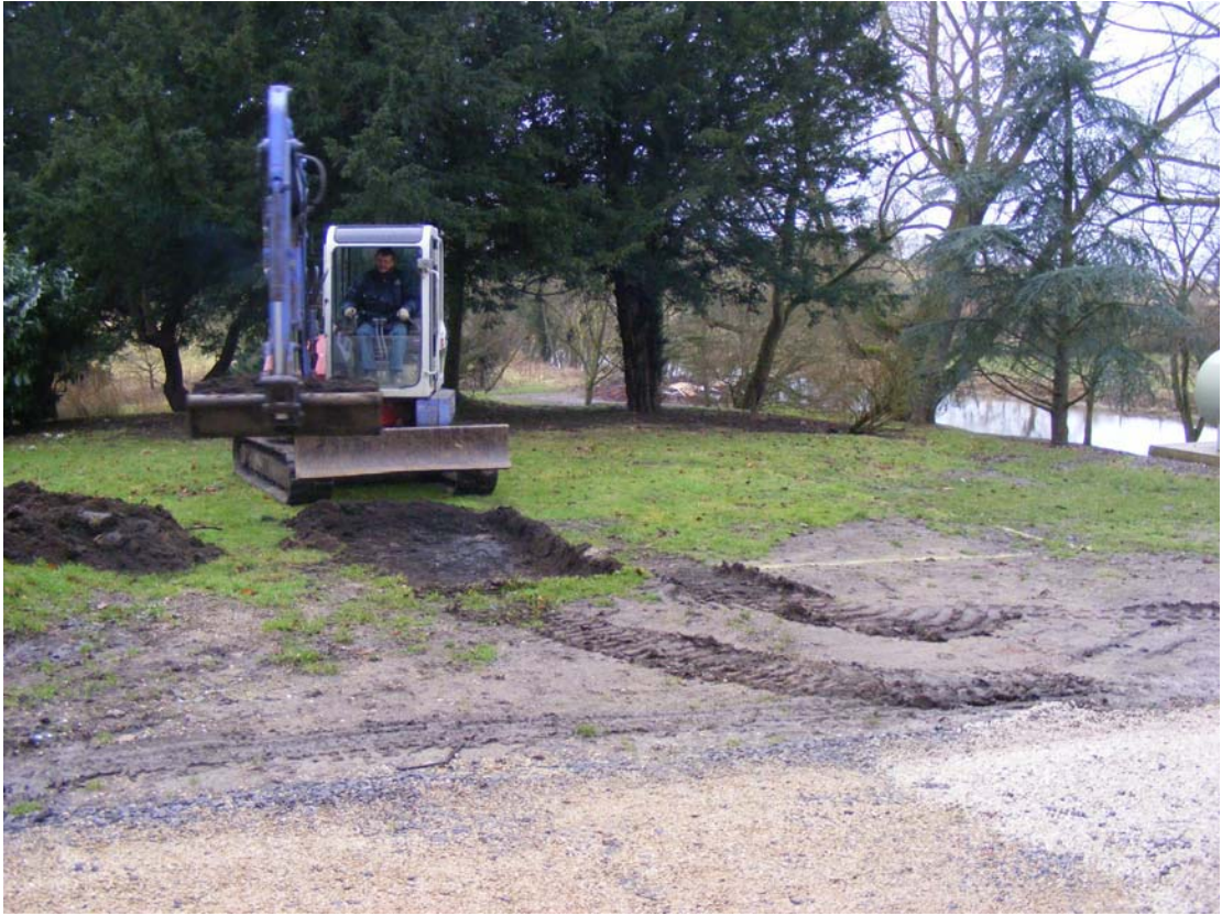
Plate 1 Excavation of Gas Tank Pit. Facing West
