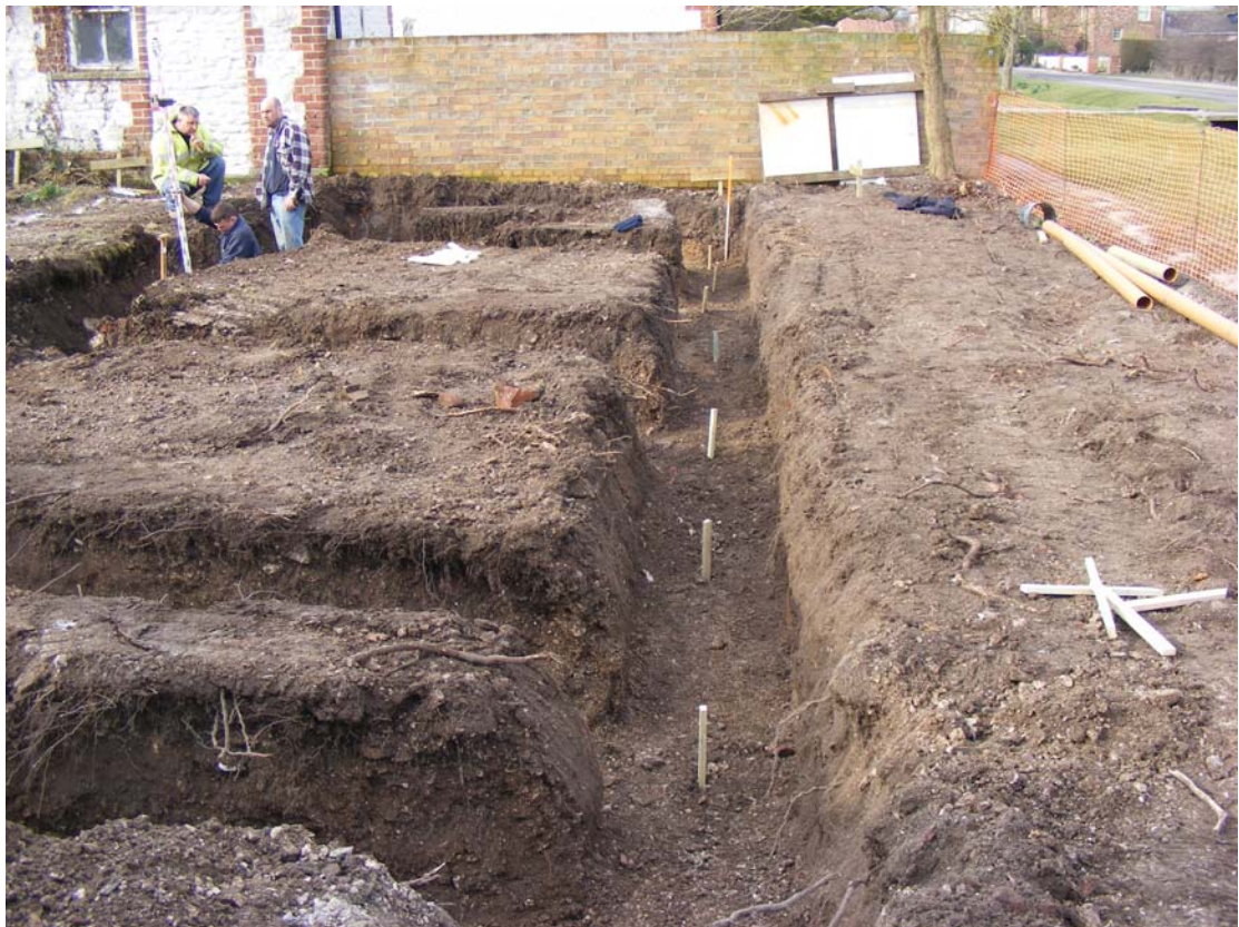
Plate 2. Foundation Trenches. Facing West
