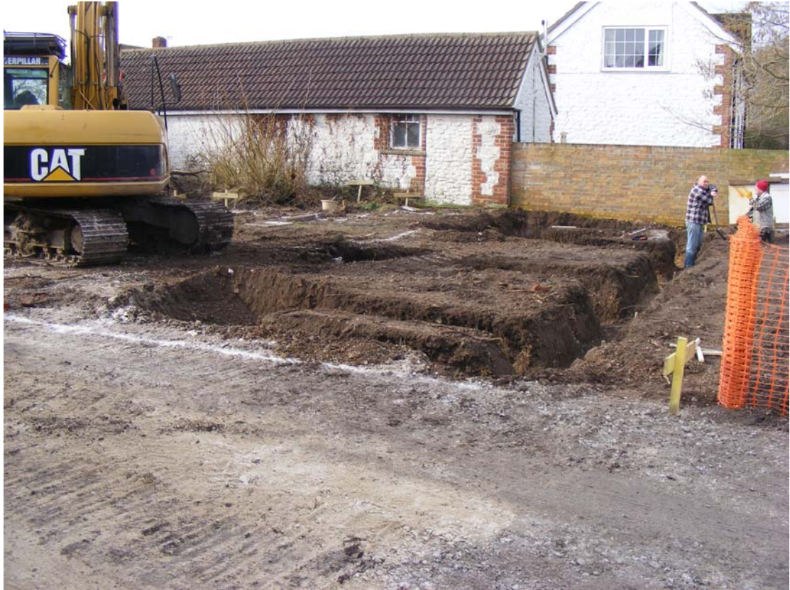
Plate 1. Excavation of Foundation Trenches. Facing South-East
