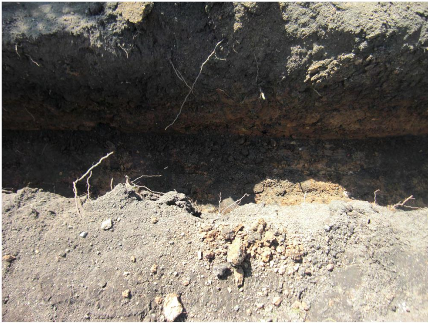
Plate 9. View of Footings.
