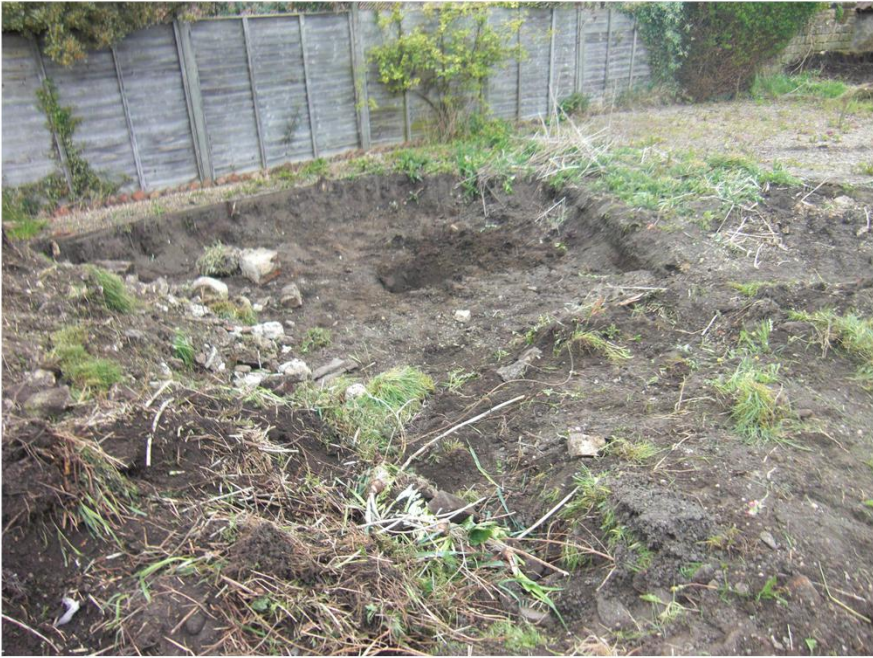
Plate 1. General View of Site. Facing South-west.
