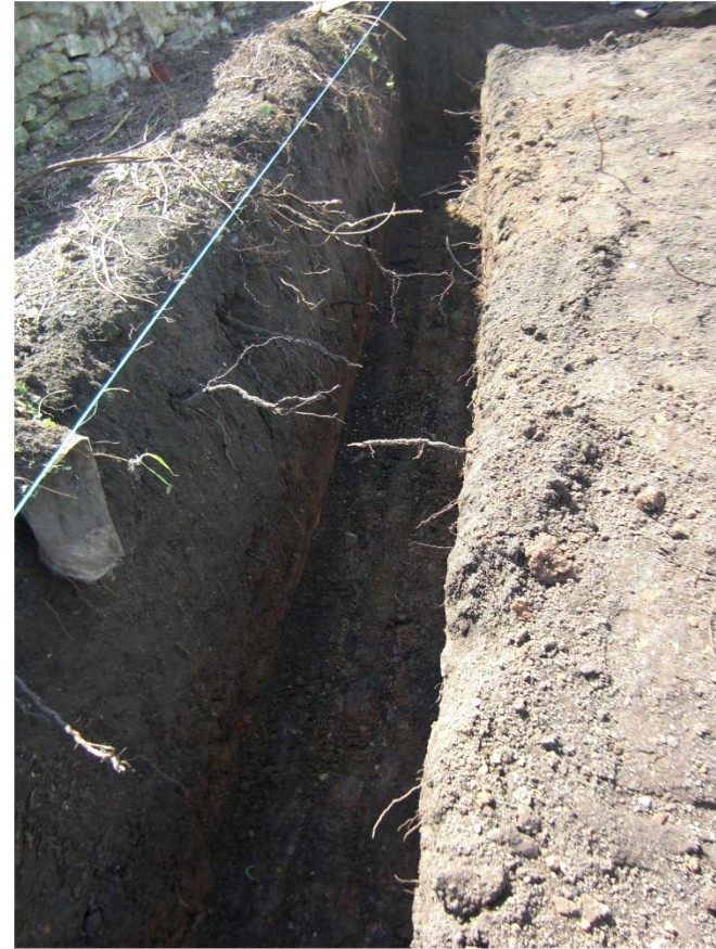
Plate 8. View of Footings.
