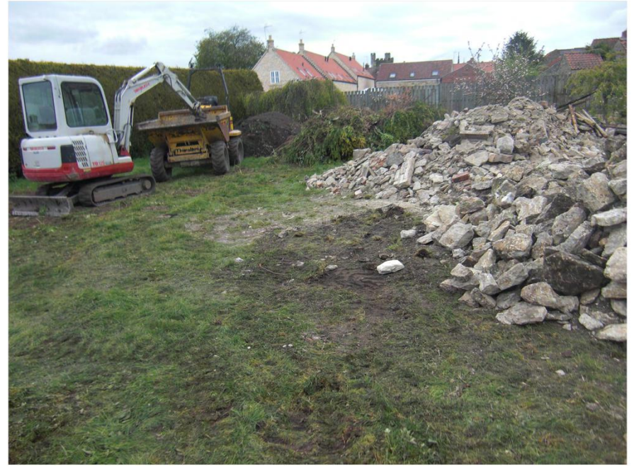
Plate 2. General View of Site. Facing West.
