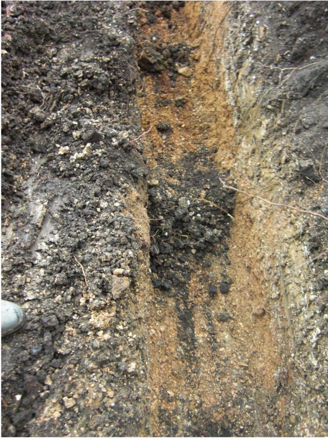
Plate 6. View of Footings.
