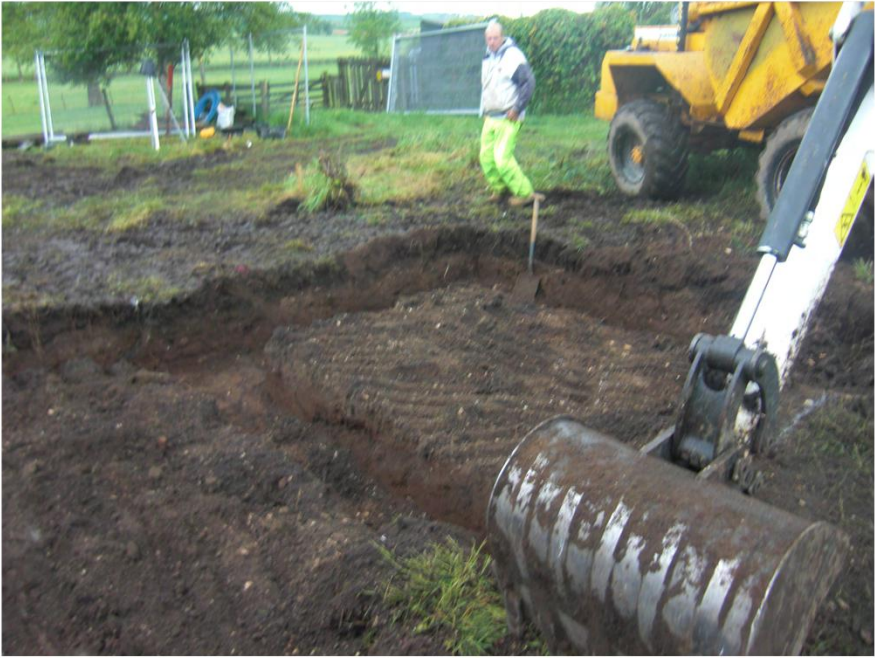
Plate 7. View of Footings.
