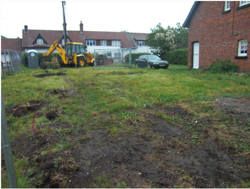
Plate 1. General View of site. Pre-excitation for footings. Facing East.
