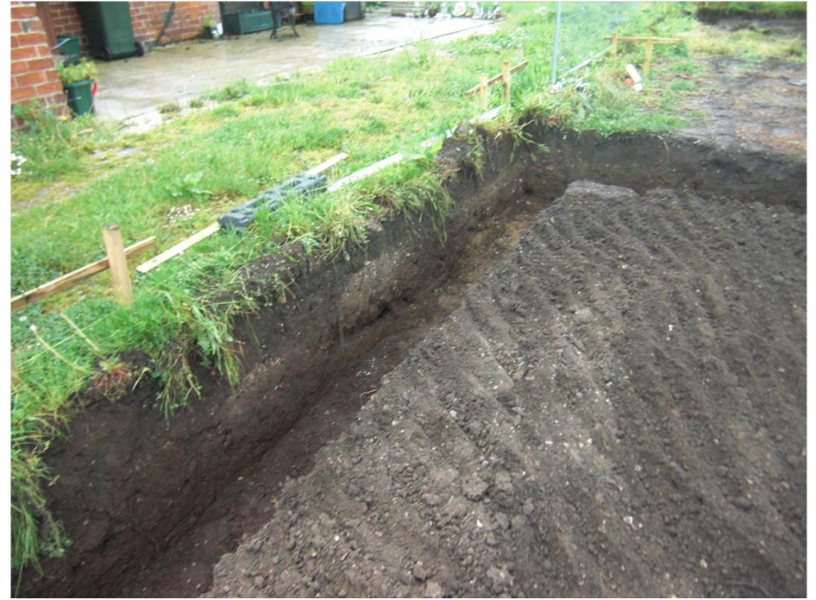
Plate 8. View of Footings.
