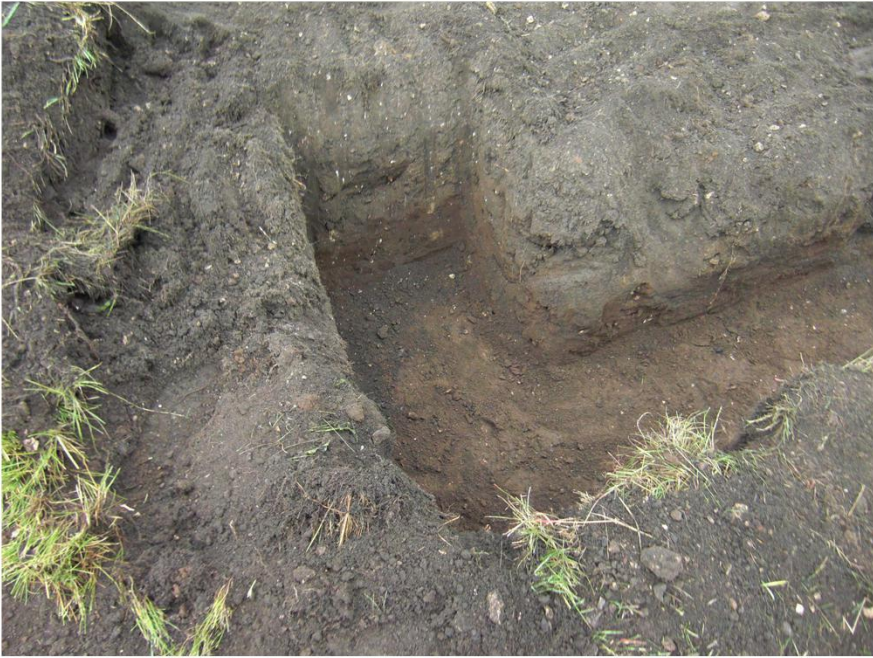
Plate 3. View of Footings.
