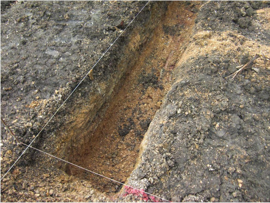
Plate 5. View of Footings.
