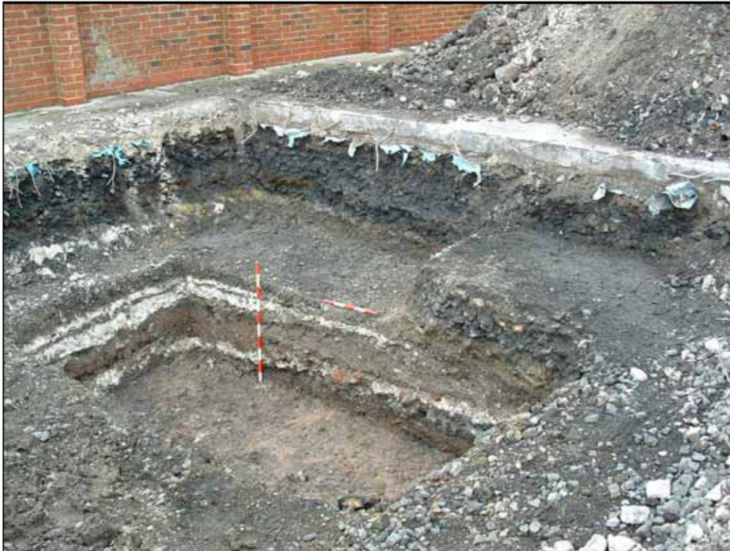
Plate 2. Trench 1 looking southwest
