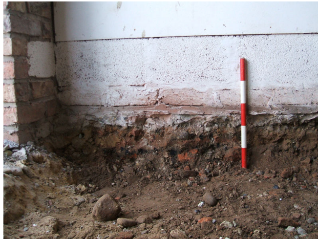
Plate 5 Make-up deposit beneath concrete floor, looking south-east
