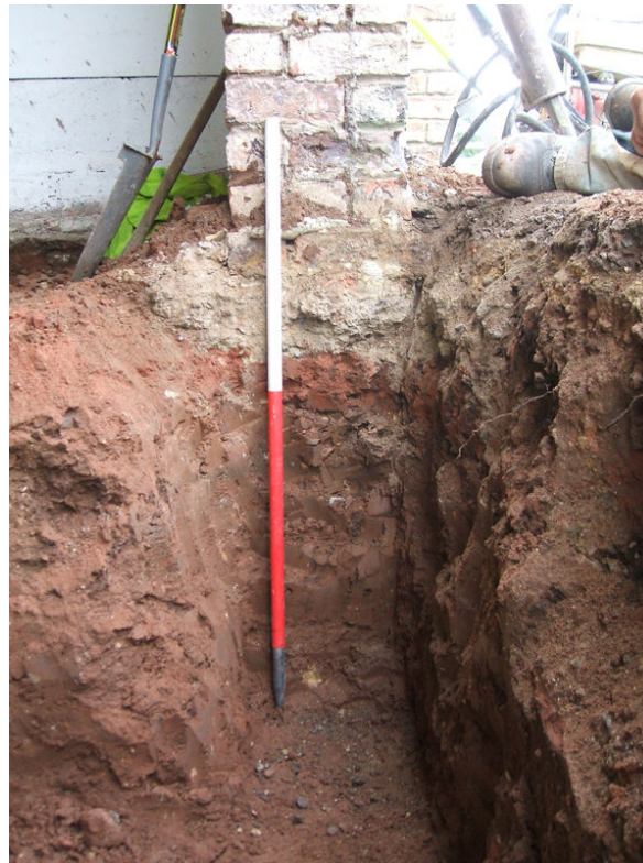
Plate 6 Foundation of doorway, looking north-west
