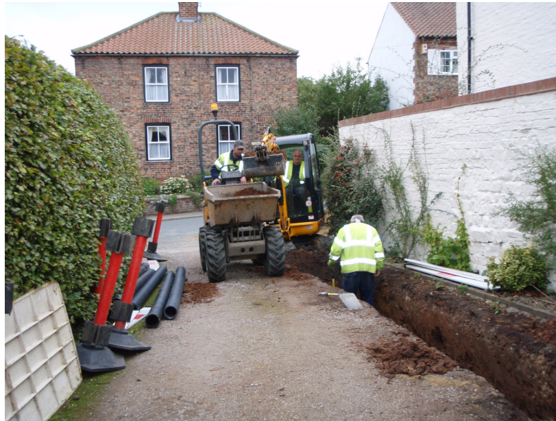
Plate 7 General view of driveway trench, looking ESE
