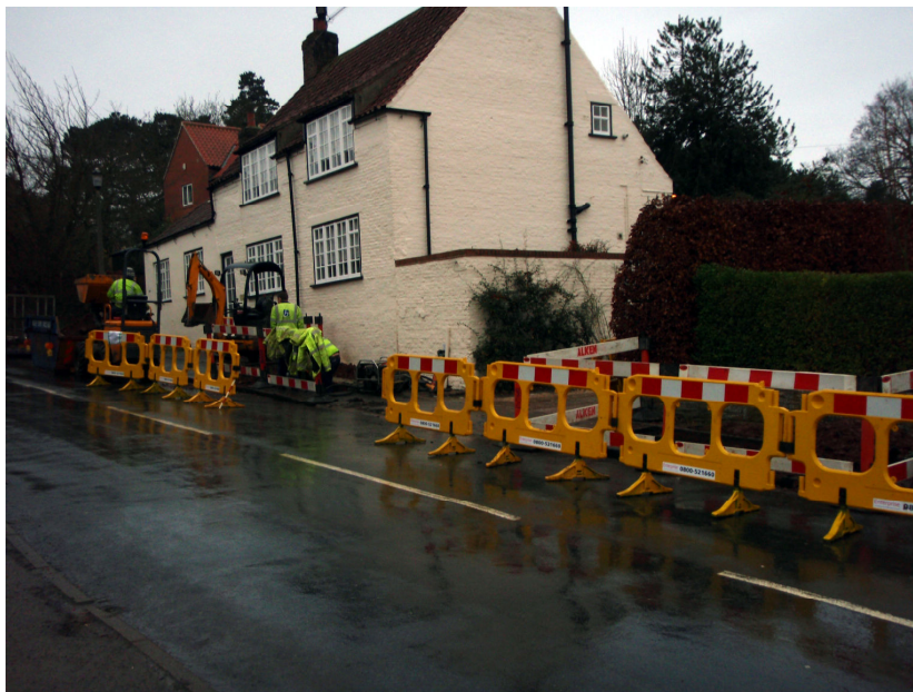
Plate 10 View of area of pavement trenches, looking SW
