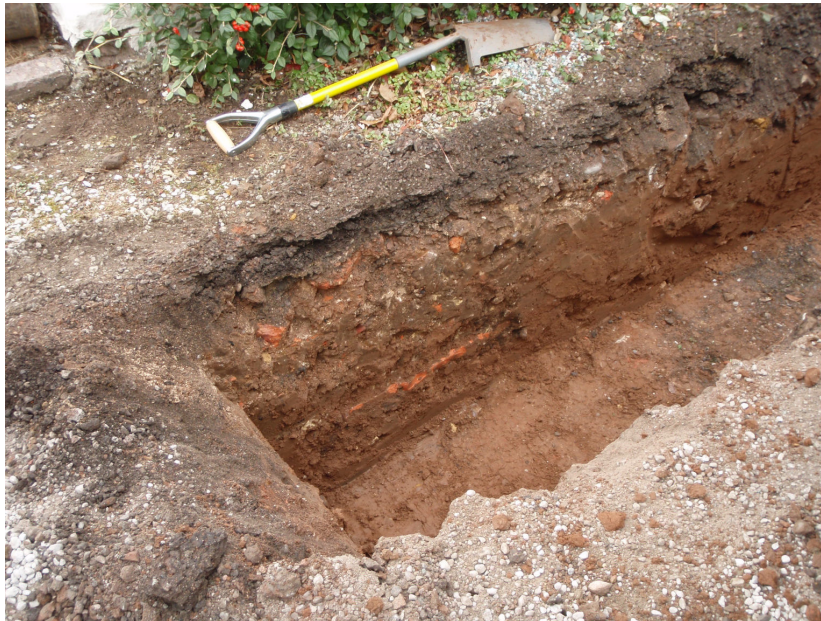
Plate 9 View of E end of driveway trench with electricity service trench to left, looking SW
