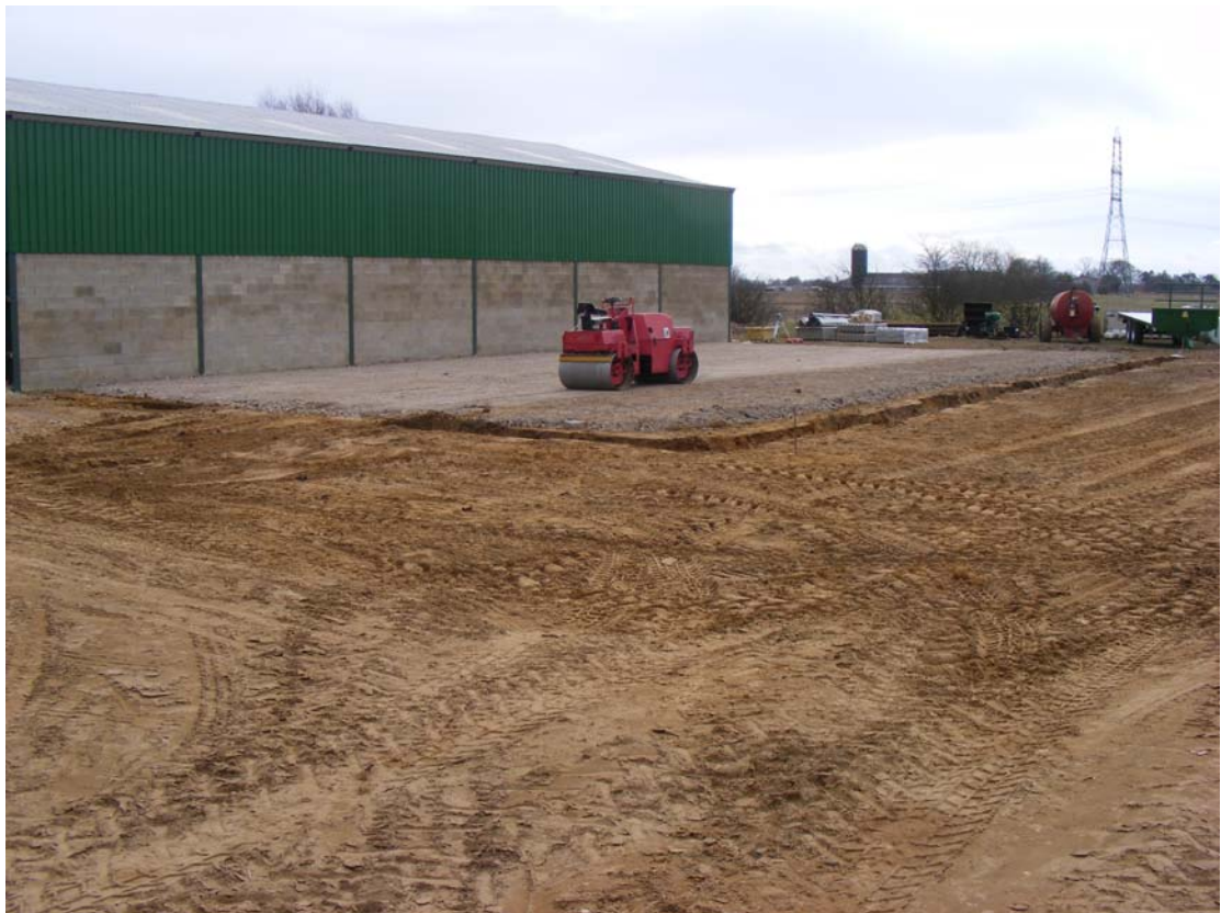
Plate 4. Post-Excavation Shot. Facing South
