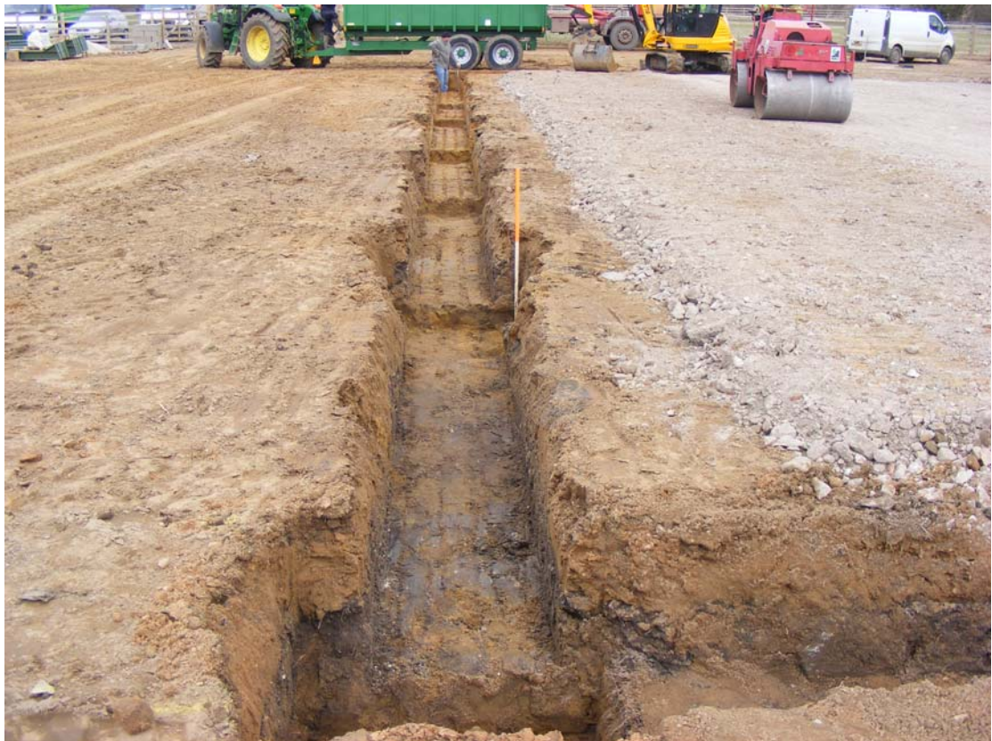
Plate 2. Foundation Trench and Stanchion Pits. Facing North-East
