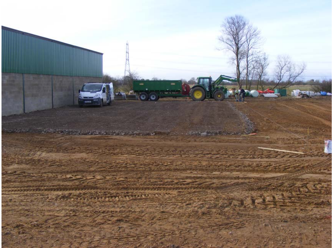
Plate 1. Pre-Excavation Shot. Facing South
