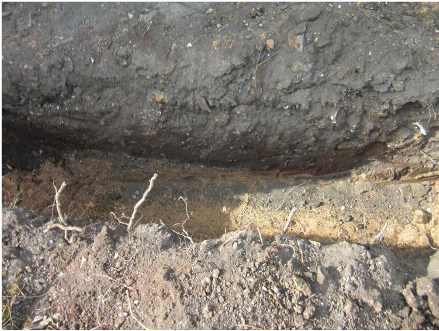
Plate 3. View of Foundation Trench.
