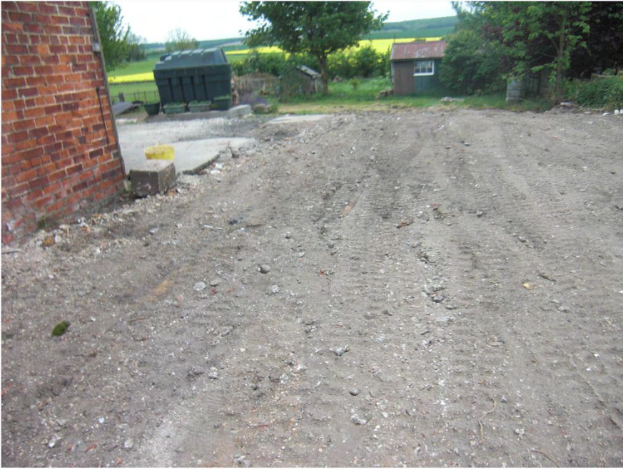
Plate 1. General View of Site. Facing East.
