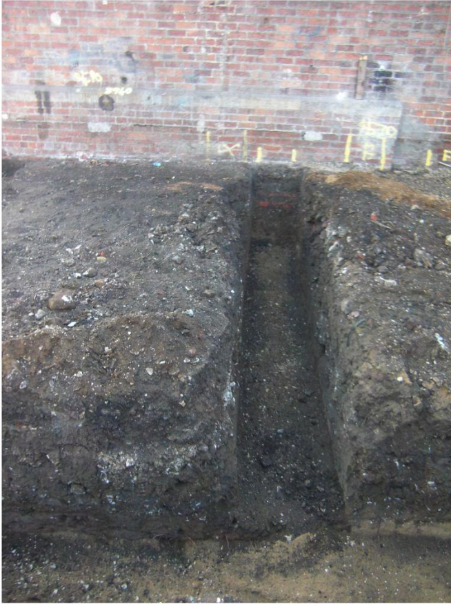
Plate 5. View of Foundation Footings. Facing East.
