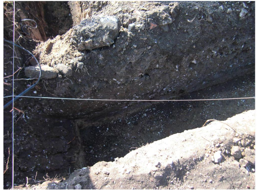
Plate 4. View of Foundation Footings.
