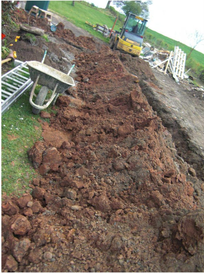
Plate 10. Section of Drainage Trench. Facing South-west.
