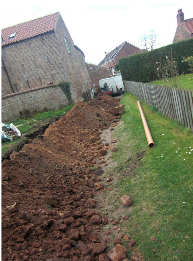
Plate 11. Section of Drainage Trench. Facing North-east.
