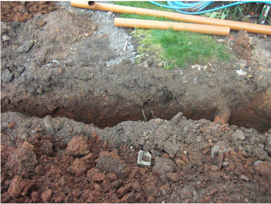
Plate 7. General Shot of Drainage Trench.
