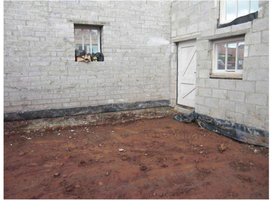
Plate 6. General Shot after removal of floor.
