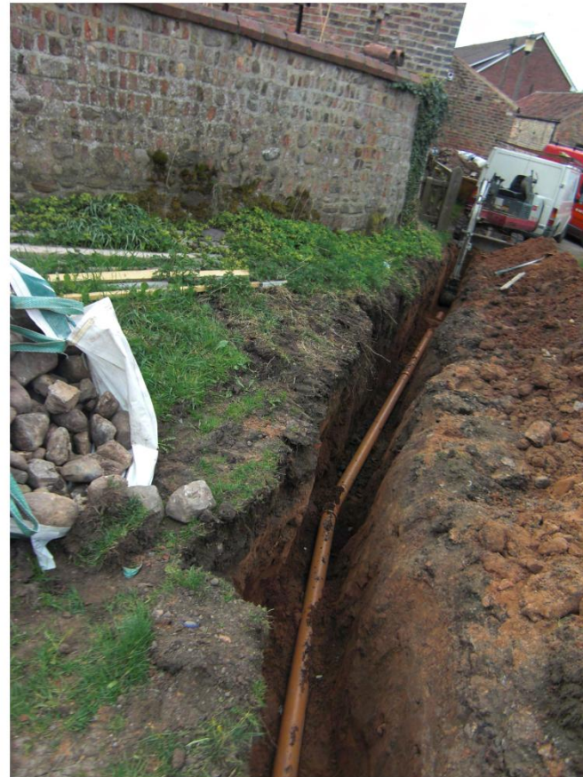
Plate 12. Shot showing length of Trench. Facing North.
