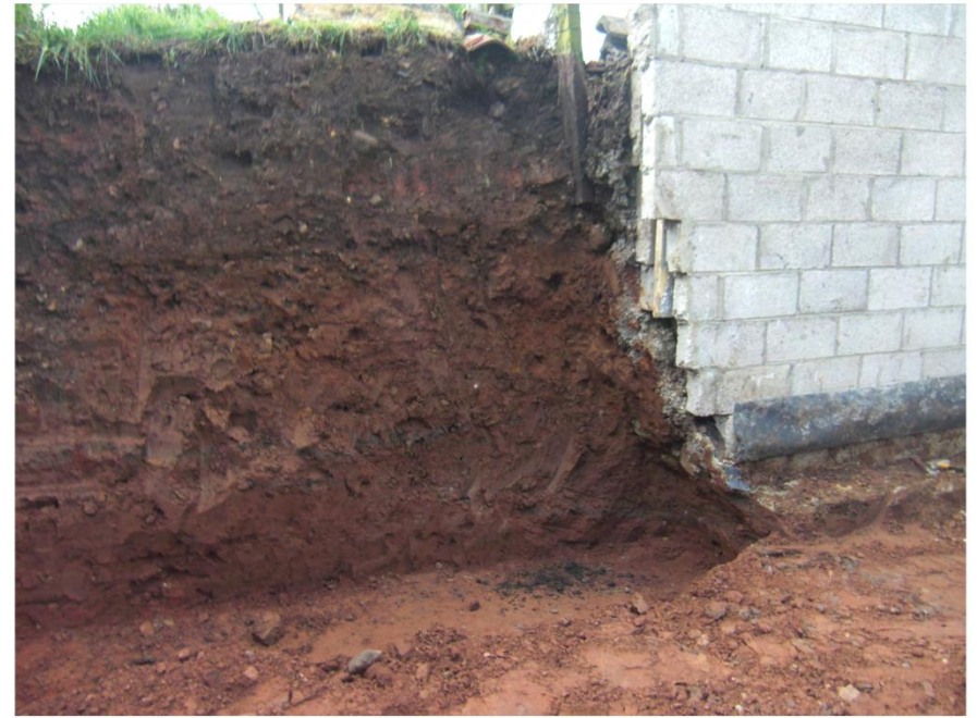
Plate 4. Section after removal of wall. Facing West.
