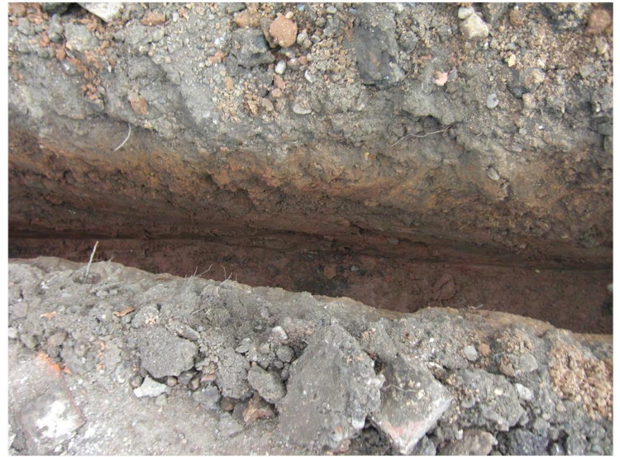
Plate 8. General Shot of Drainage Trench.
