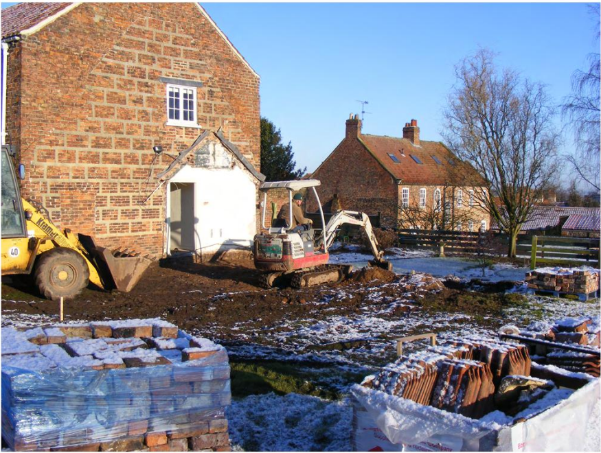
Plate 1. Excavation of Foundation Trenches. Facing North-east.
