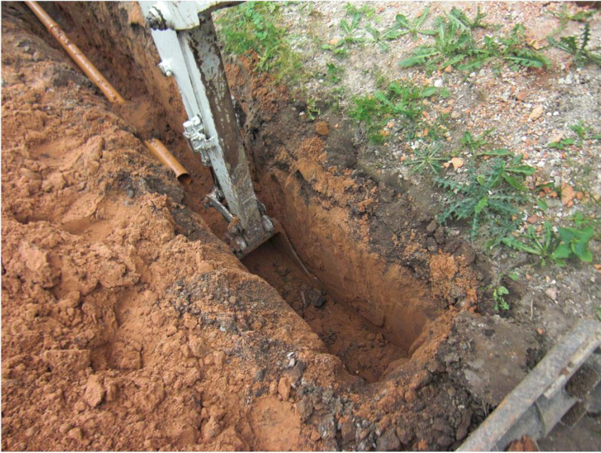
Plate 9. Section of Drainage Trench.
