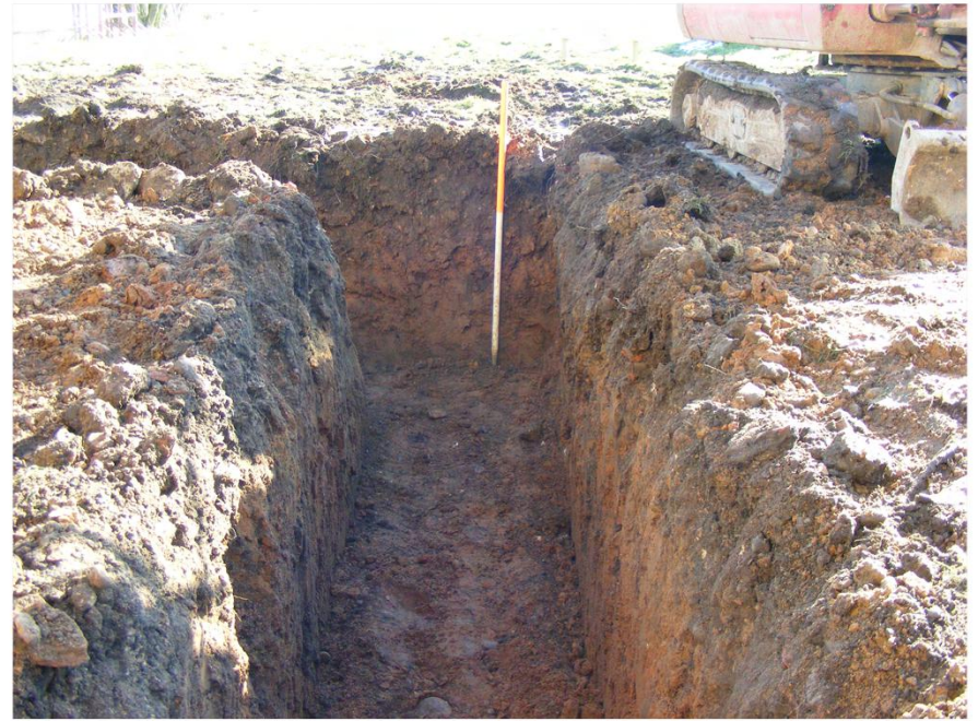
Plate 2. Excavated Foundation Trench. Facing South-west.
