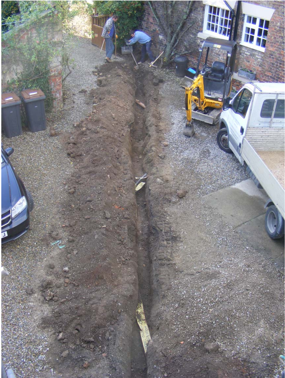
Plate 2. Overall View of Service Trench. Facing South-West
