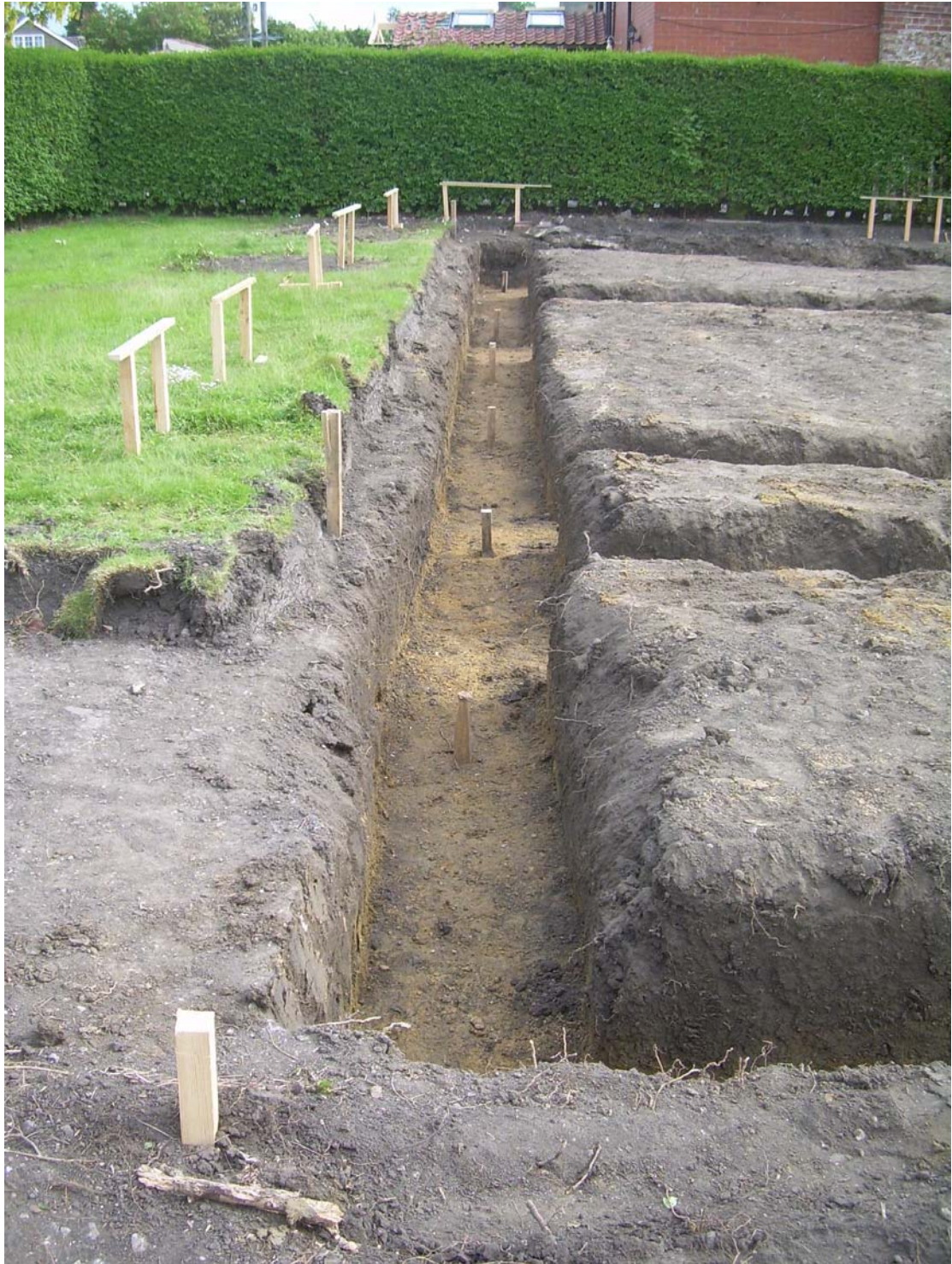
Plate 6. Detail of Strip Foundations. Facing South.
