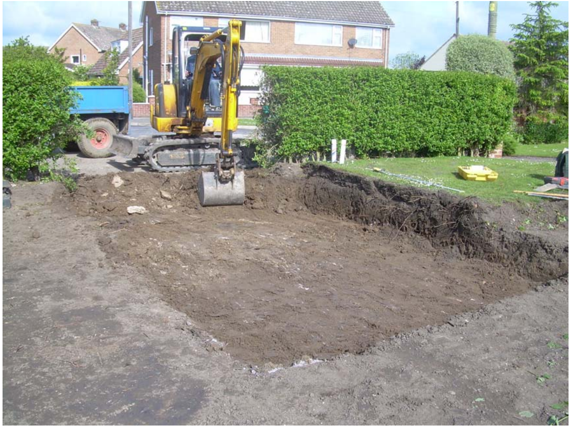
Plate 3. Site Entrance after stripping. Facing North-east.
