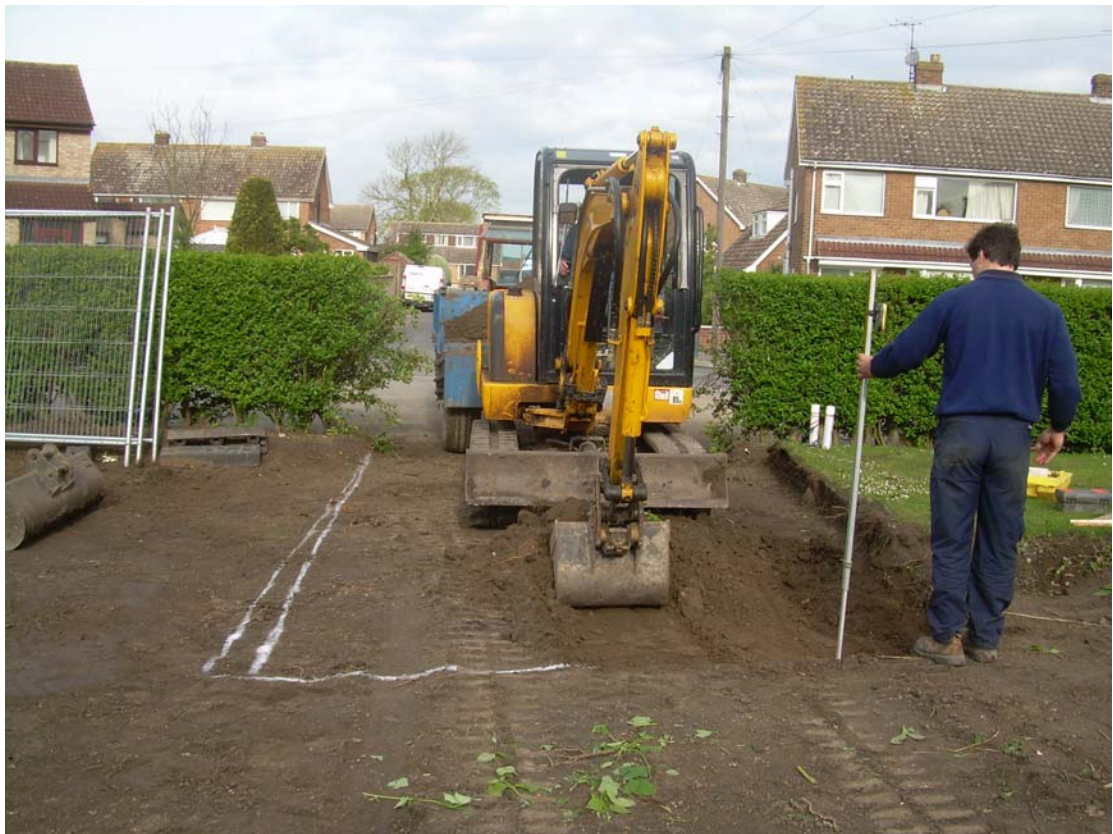
Plate 2. General view of Site entrance. Facing West.
