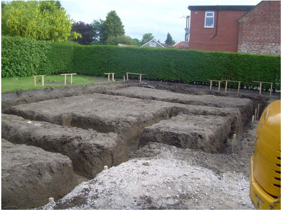
Plate 5. Strip Foundations after excavation. Facing South-east.
