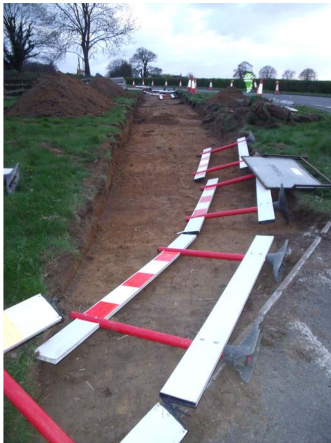
Plate 2. Area 1, Layer [3], looking South-West (along corridor for new footway)
