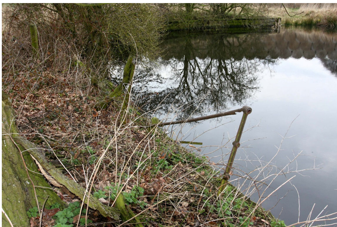
Plate 10 Pond 3 detail of iron railing with later wooden post to top left, looking E
