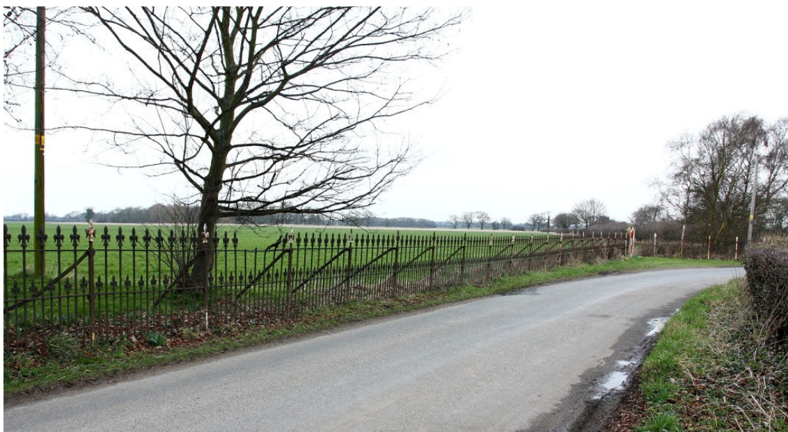
Plate 12 Park railings, looking NNE
