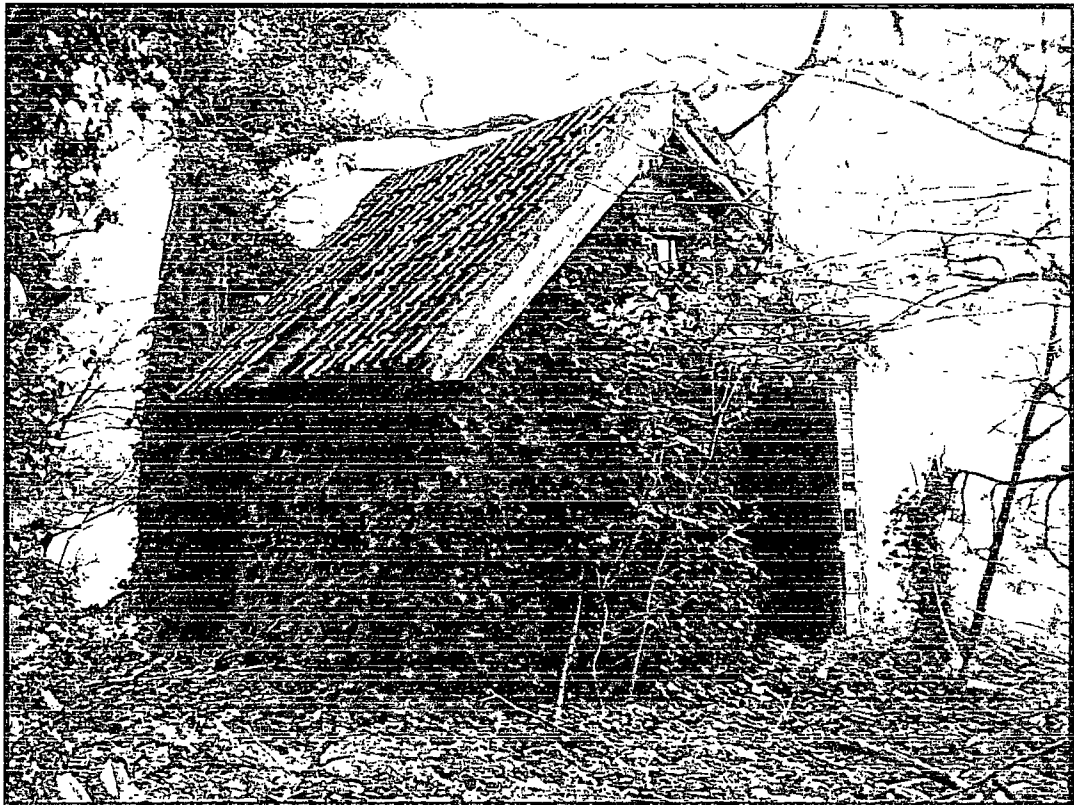
Plate 4 : Garden shed from south
