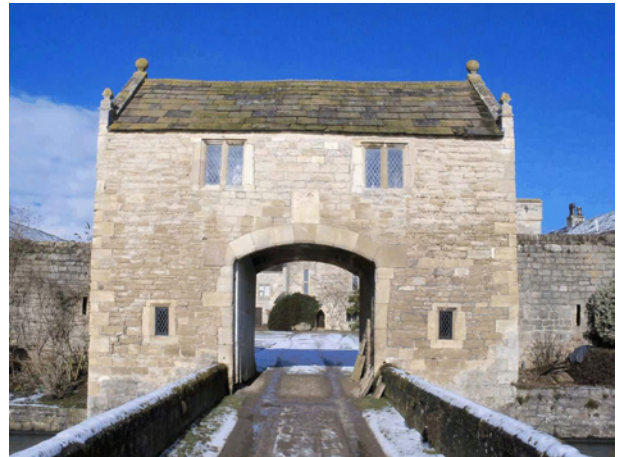
Plate 1 Markenfield Hall gatehouse south elevation
