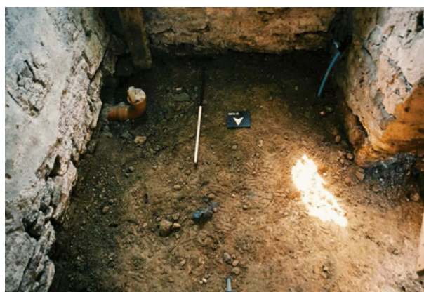
Plate 4 Ground floor of gatehouse following ground reduction
