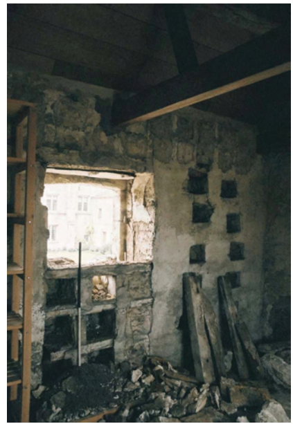
Plate 5 Window opening created from blocked doorway showing nest boxes (Scale 1.0m)
