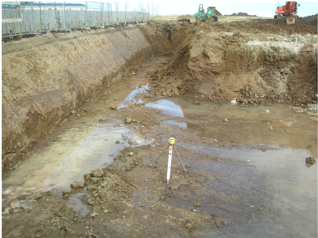
Plate 6 The pumping station excavation in progress, looking east
