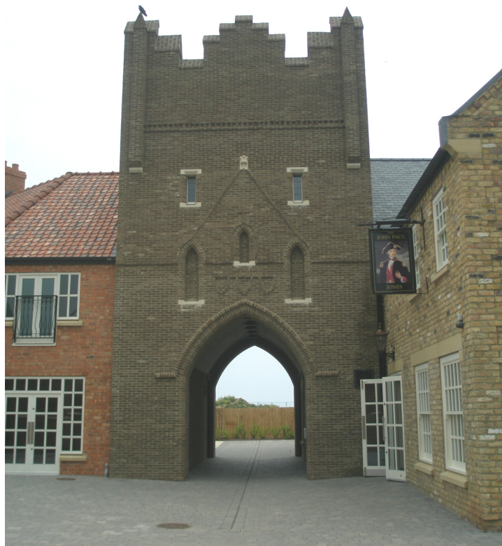
Plate 10 The replica of the North Bar, Beverley, viewed from the south-west
