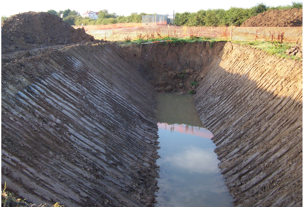
Plate 2 The diverted open drainage channel, looking south
