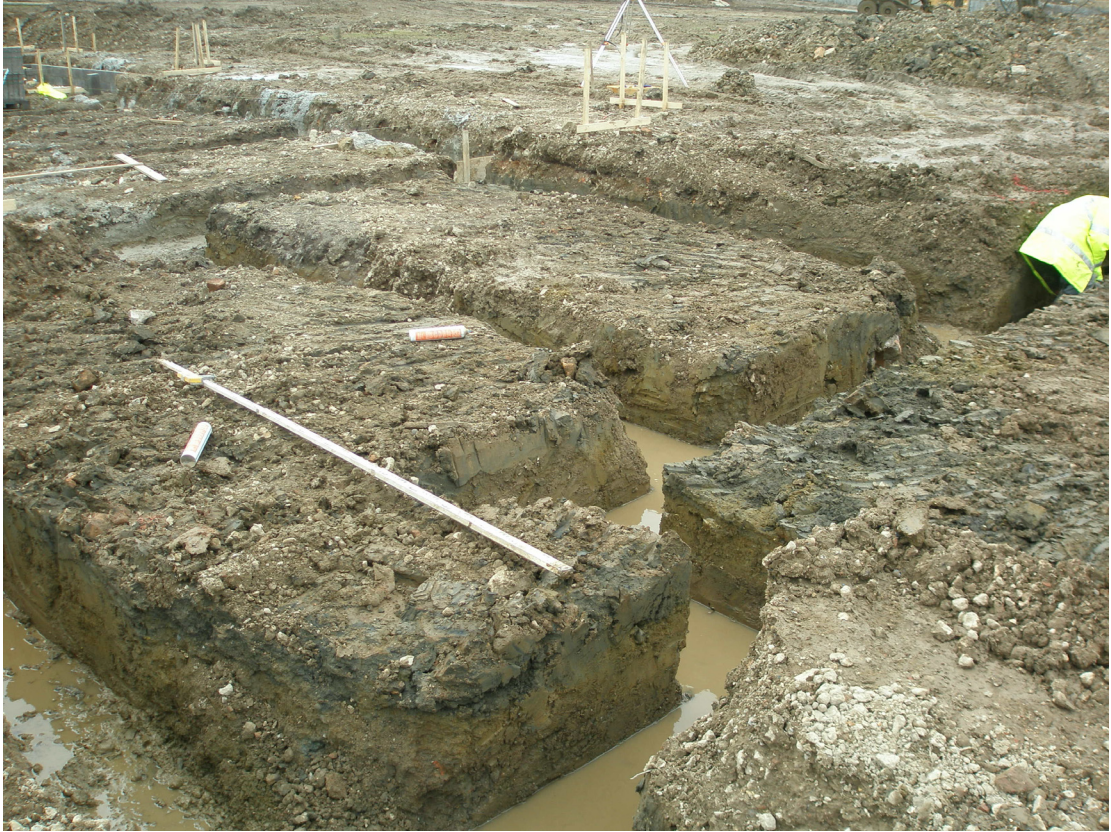
Plate 7 Foundation trenches for plots 39 and 40, looking north-west
