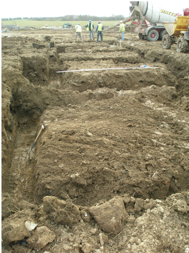
Plate 9 Foundation trenches for plots 62-64, looking south-west
