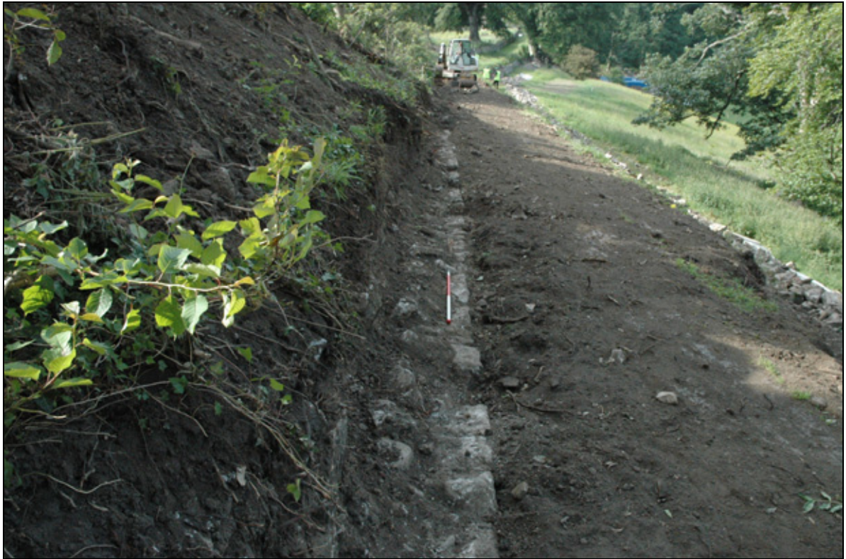
Figure 3: footings for upper retaining wall, looking south
