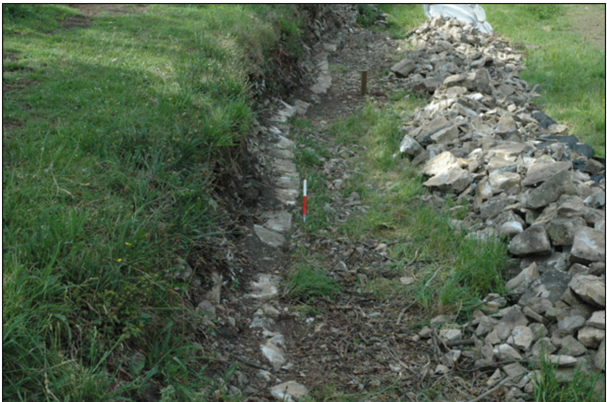
Figure 4: footings for lower retaining wall, looking south
