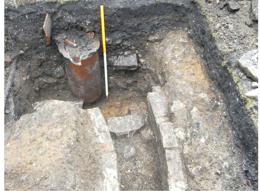
Plate 4. Trench 1: Drain Culvert 1007 and Soakaway Pit 1010. Facing South.
