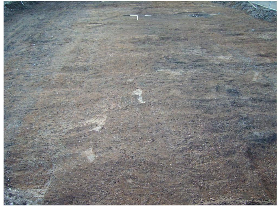
Plate 2. Site after cleaning. Facing West.
