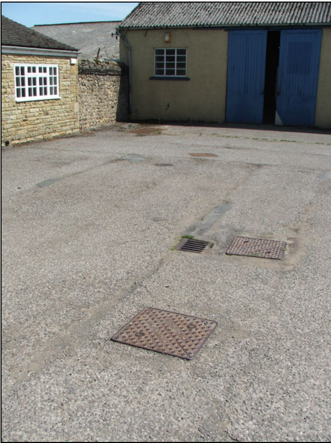
Plate 3. Services and drainage in the forecourt
