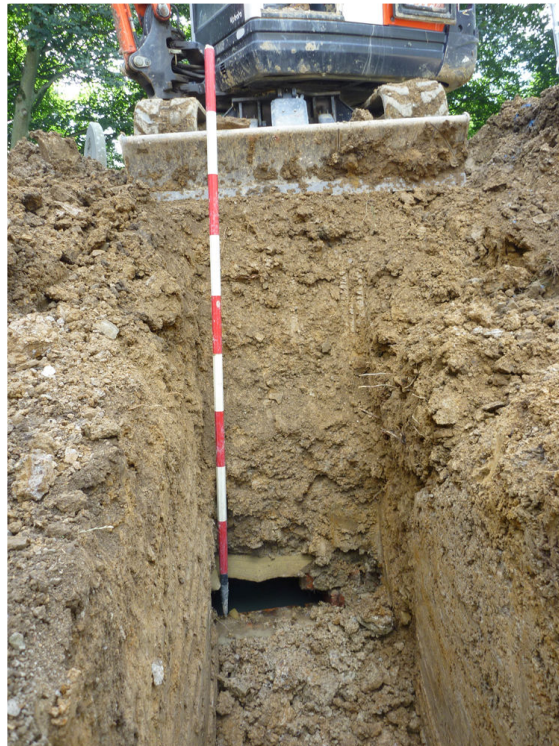
Plate 3 First encounter with brick-built vault, looking south-west
