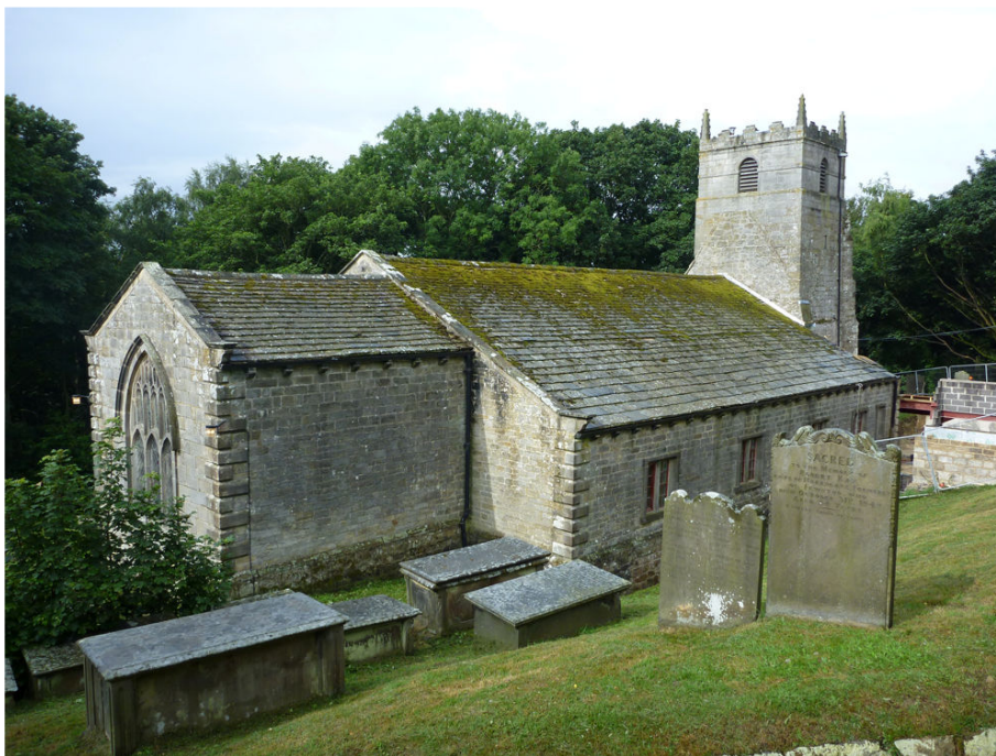
Plate 1 Church from north-east, showing slope of graveyard
