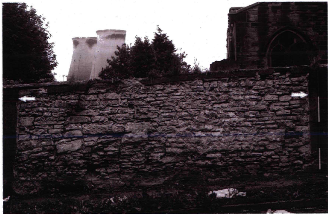
Plate 6. Wall section 106 facing west. Arrow indicates height aOD of 21.55m
