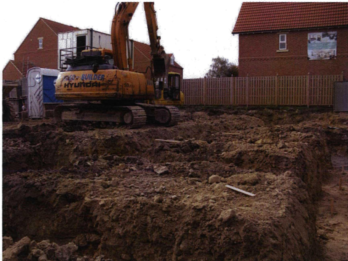
Plate 6 Plots 14 through 17 overall, looking southwest.
