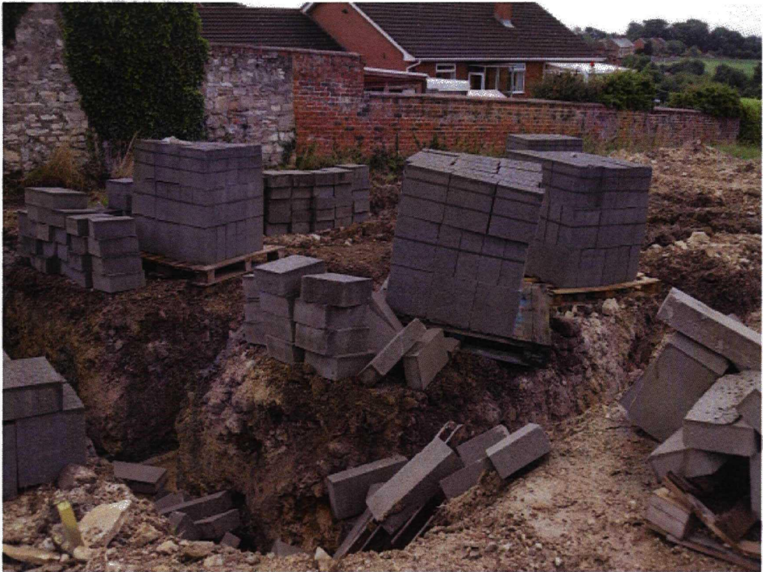
Plate 3 Plot 13, viewed from the northwest.
