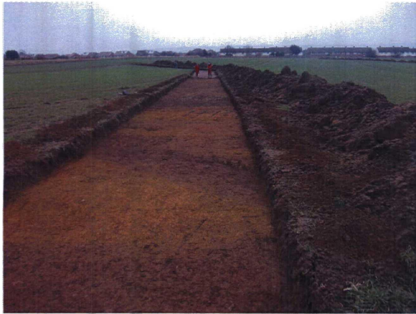
Plate 27. General View of Trench 43. Facing South.
