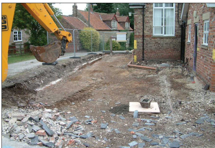
Photo 1: View of site following initial ground-strip, looking east.
