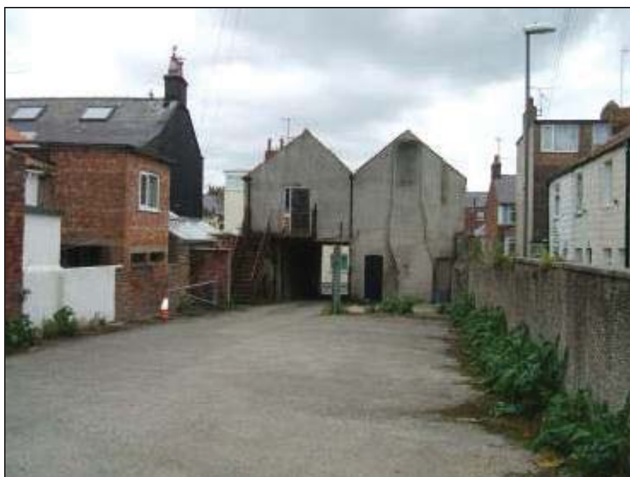
Plate 10 Current main access to site, looking south-south-west
