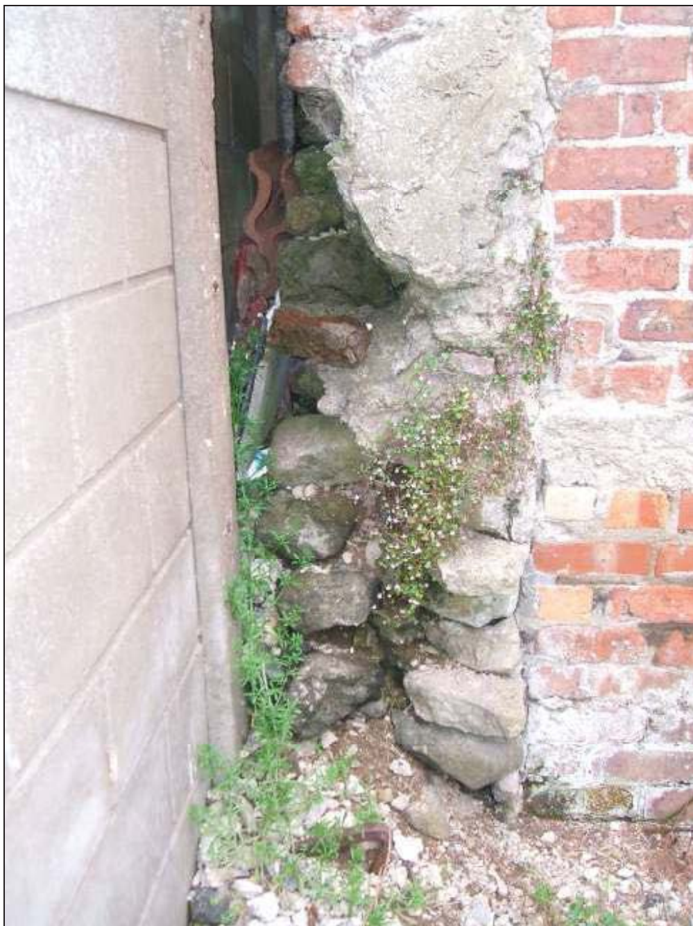
Plate 8 Detail of stone walling in possible fish-curing structure, looking north-north-east
