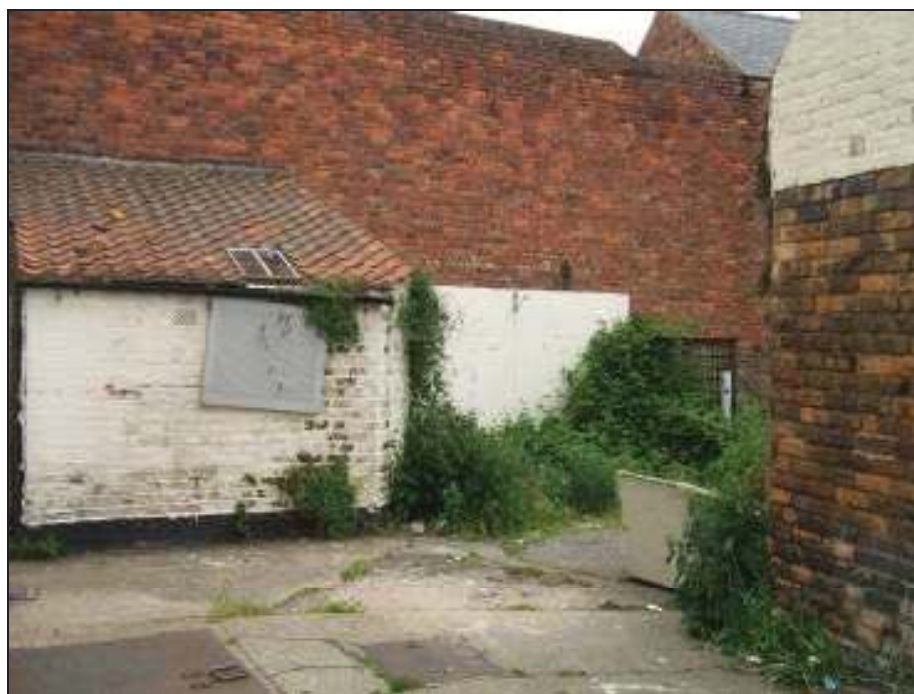
Plate 12 Part of yard to rear of Crown Hotel, looking south-east
