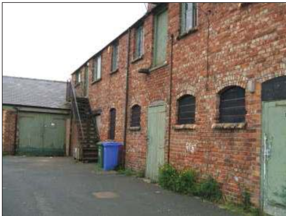
Plate 9 Brick range, possibly stables or workshops, in central part of site, looking south-west
