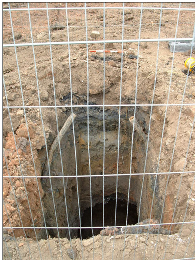
Plate 2. North-facing section Trench D
