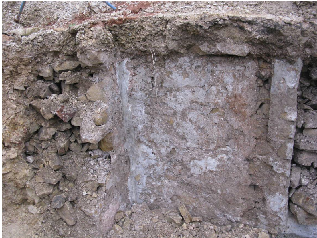
Plate 9 Showing detail of partially faced limestone with light blue grey plaster for cellar wall (403). Looking north.
