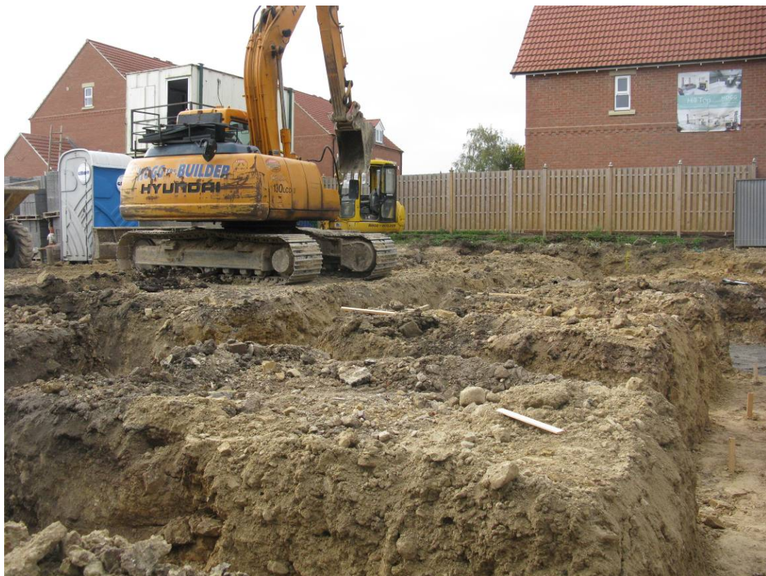
Plate 6 Plots 14 through 17 overall, looking southwest.
