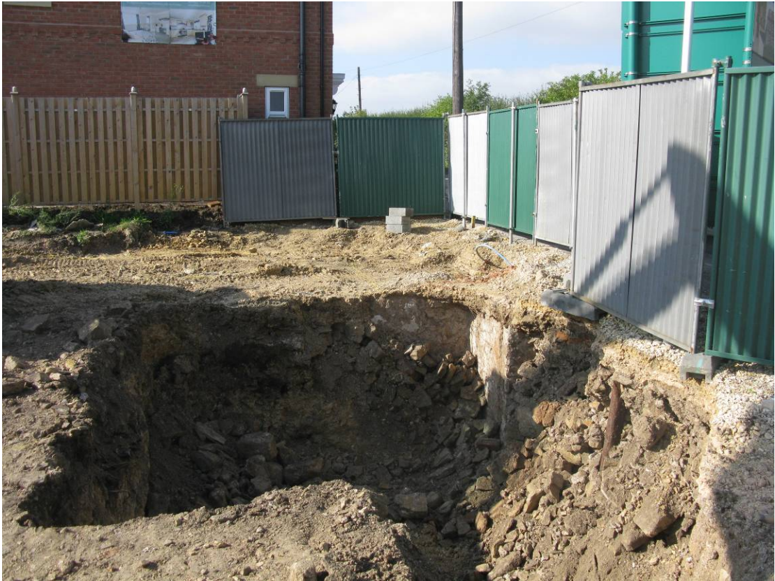
Plate 7 Former farm cellar (403), looking west.
