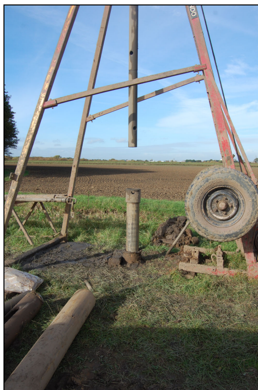
Plate 4: Borehole 10 during excavation
