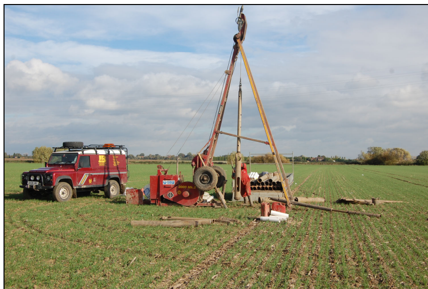
Plate 1: Borehole 1 during excavation
