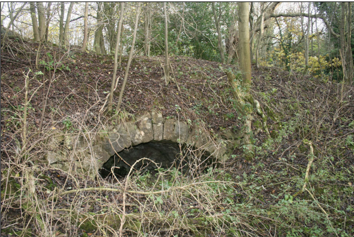
Plate 15. The draw arch of Kiln E. Lower part of kiln is backfilled
