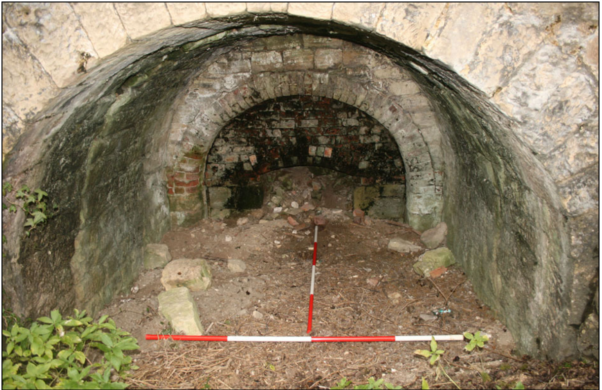
Plate 9. Detail of the draw arch and draw hole
