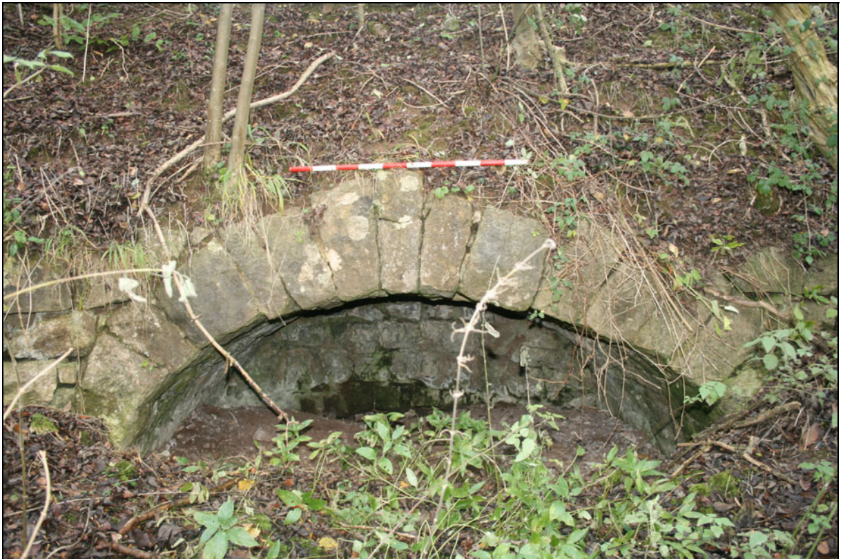
Plate 16. The draw arch and draw hole of Kiln E
