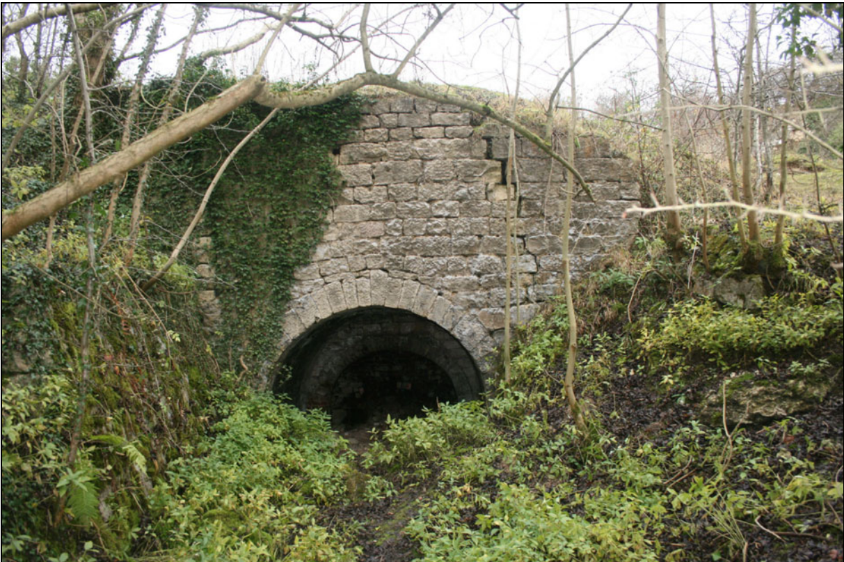
Plate 8. General view of the facade of Kiln C
