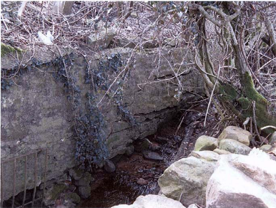
Figure 16: Ditch along part of the eastern boundary
