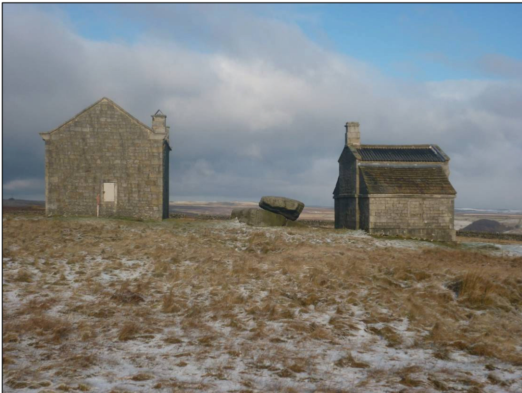
Plate 2: South elevations of house and Rocking Hall, with Rocking Stone between, looking N.
