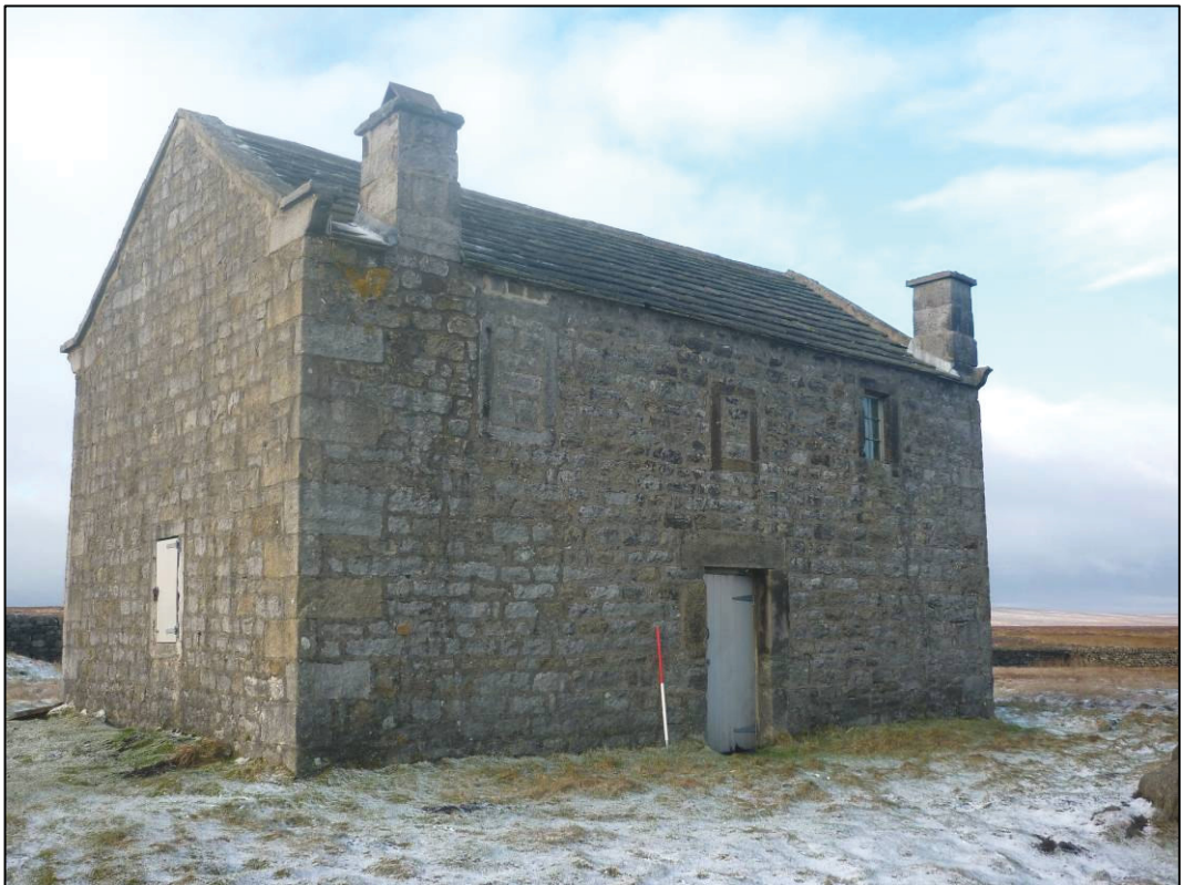
Plate 9: South and east elevations of house, looking NW.
