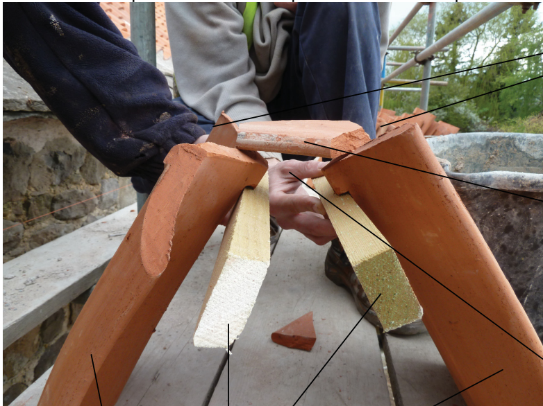
Plate 11 Example: the creation of potential bat roost spaces under ridge tiles (cross-section)
