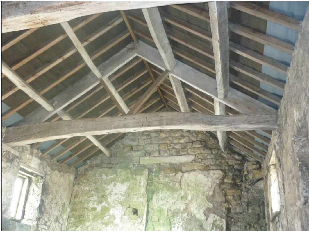
Plate 12: North roof truss in house, looking N.
