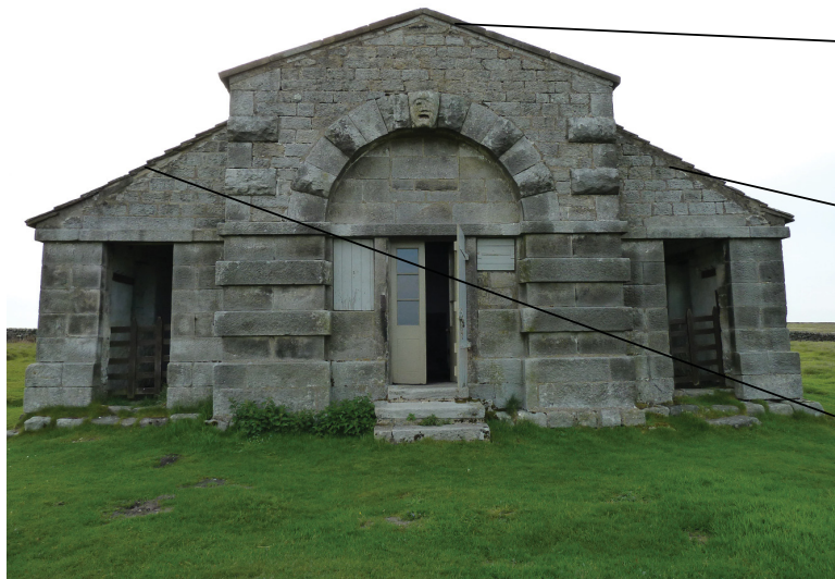
Plate 2 South elevation: gaps suitable for bat entry into potential roosts between overlapping stone slates
