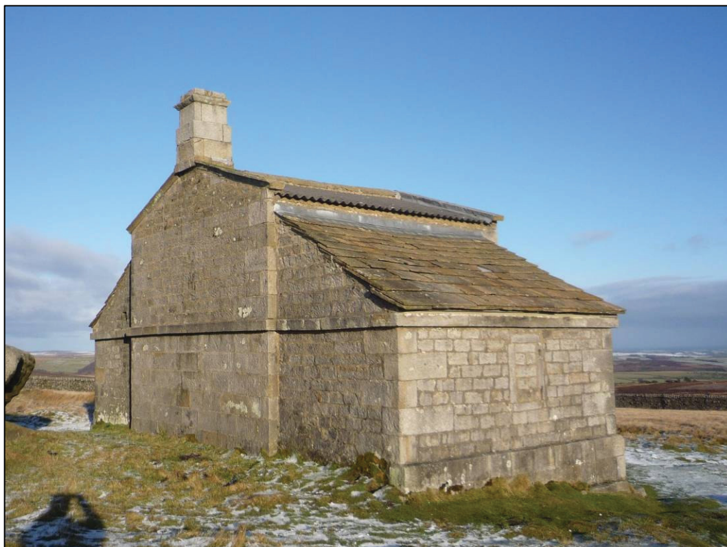
Plate 5: South and west elevations of Rocking Hall, looking NE.
