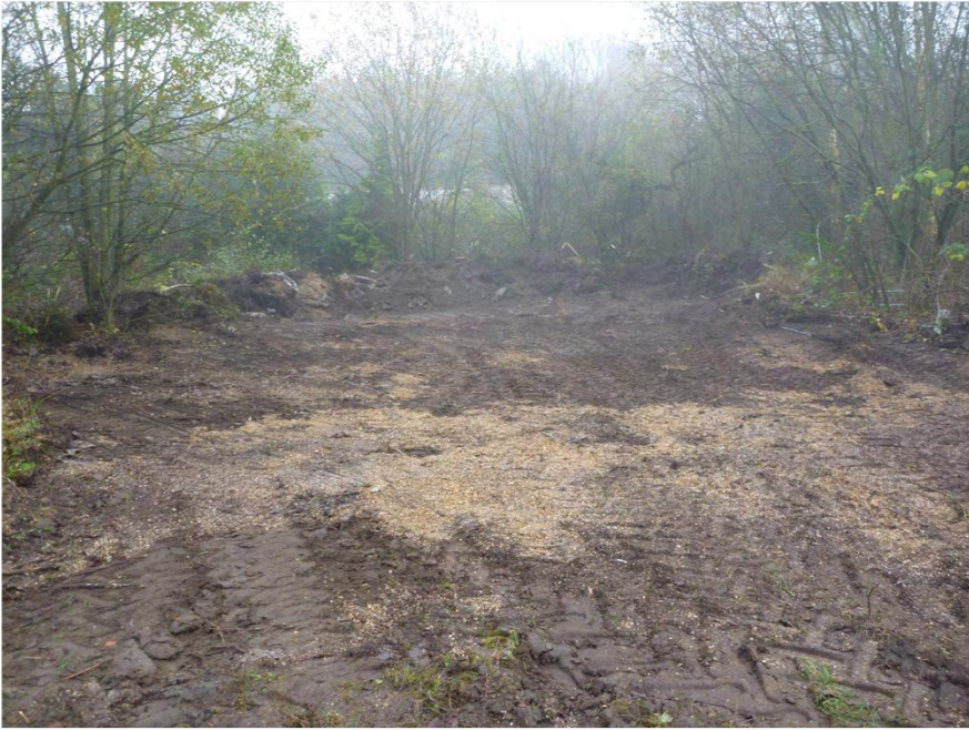
Plate 15. Trench 4. Post vegetation clearance. Facing West.
